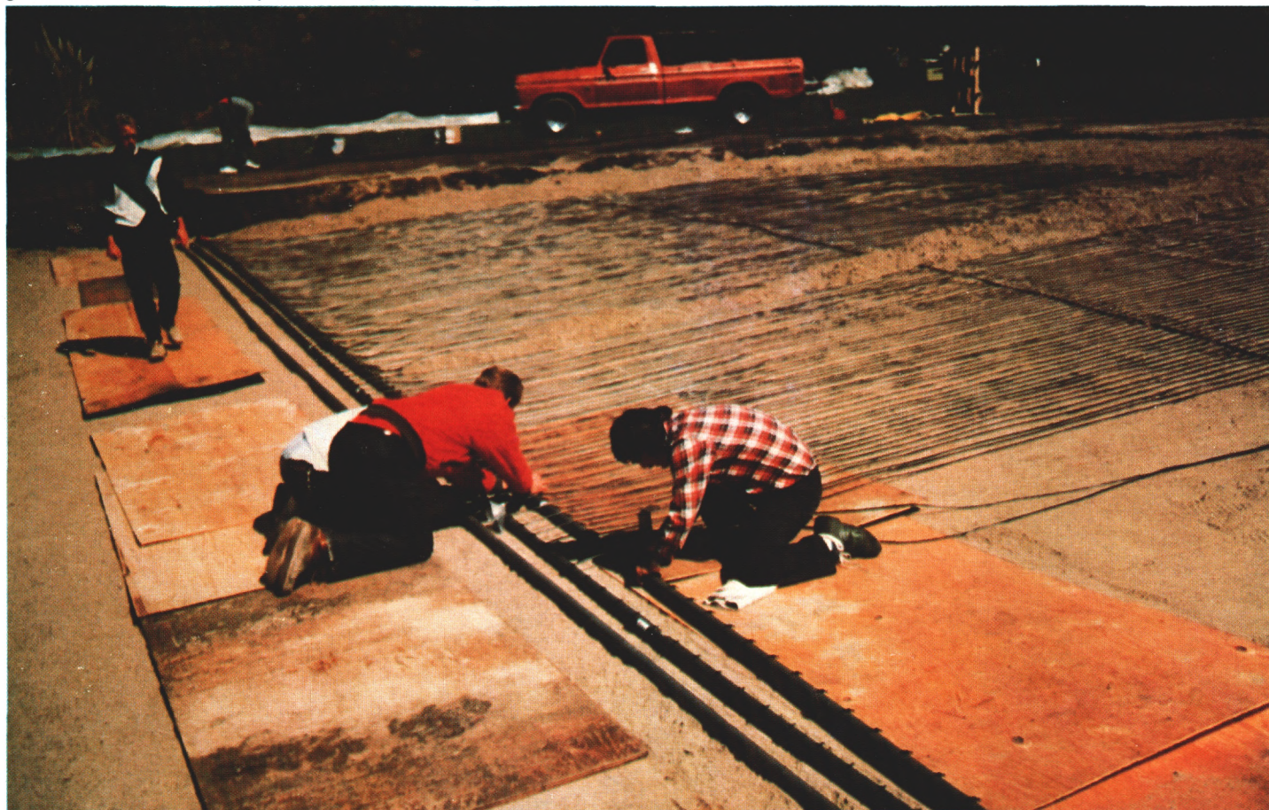
Stay alive at 55°. A constant soil temperature will be maintained year round on the 5th green with the installation of the sub-surface heating systems.
