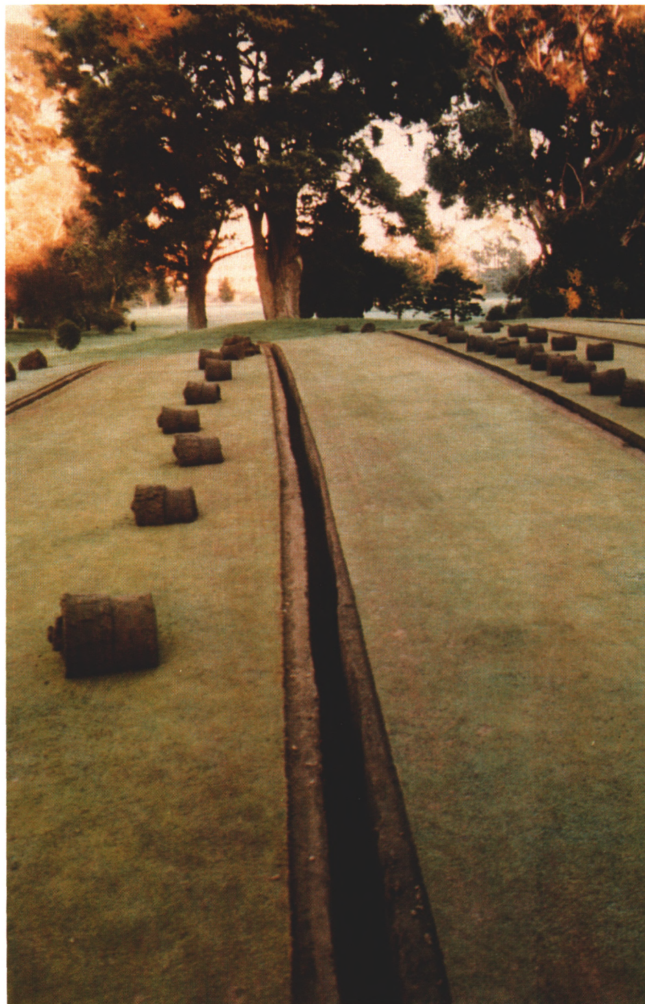
Correcting drainage problems on greens has become more important with increased playing pressures. Installing a trench and backfilling with materials that provide good water conductivity is one corrective technique used to improve drainage.
