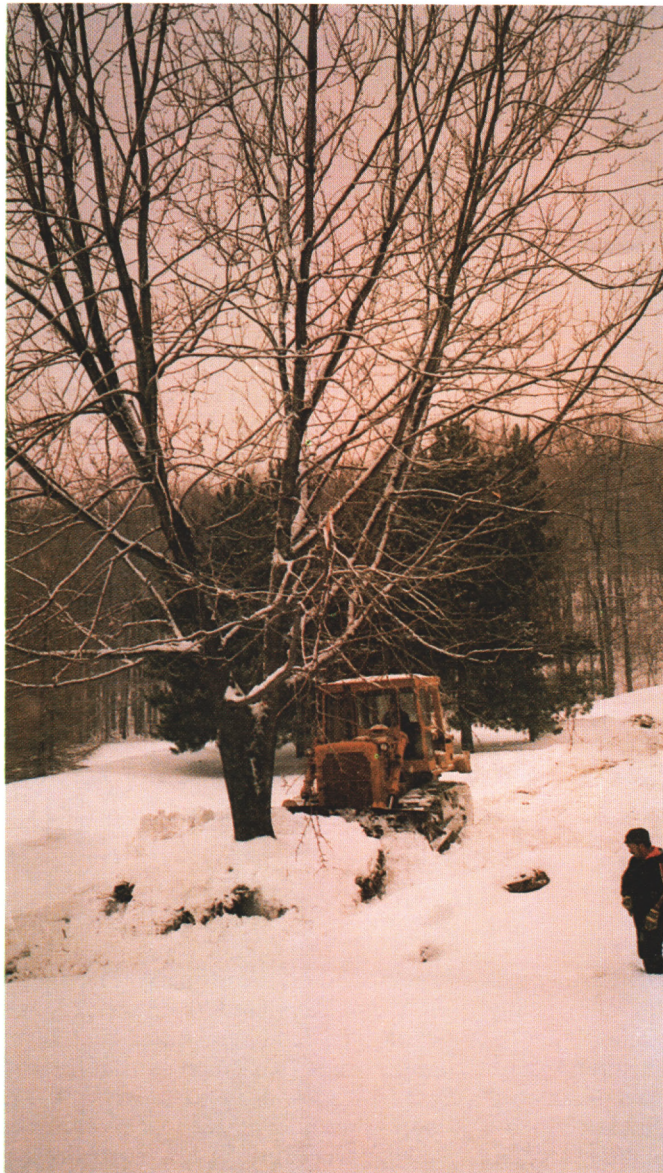
(Left) Moving the transplant trees is accomplished during the winter, after the ground has frozen thoroughly. A D-8 class dozer is required to move larger trees.
