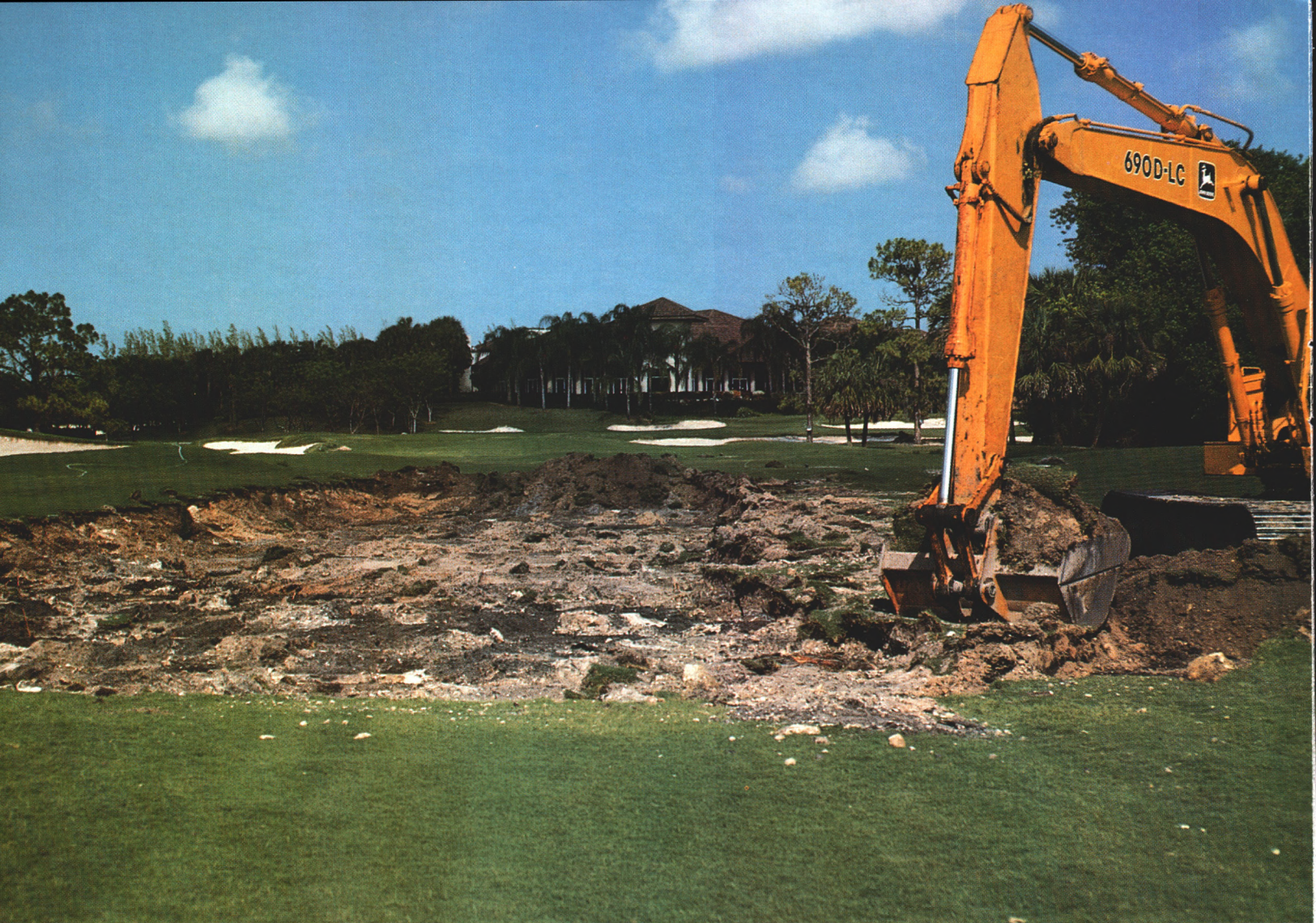
Fairway excavation removed the coral rock and muck soil pockets that previously hindered water percolation through the soil.
