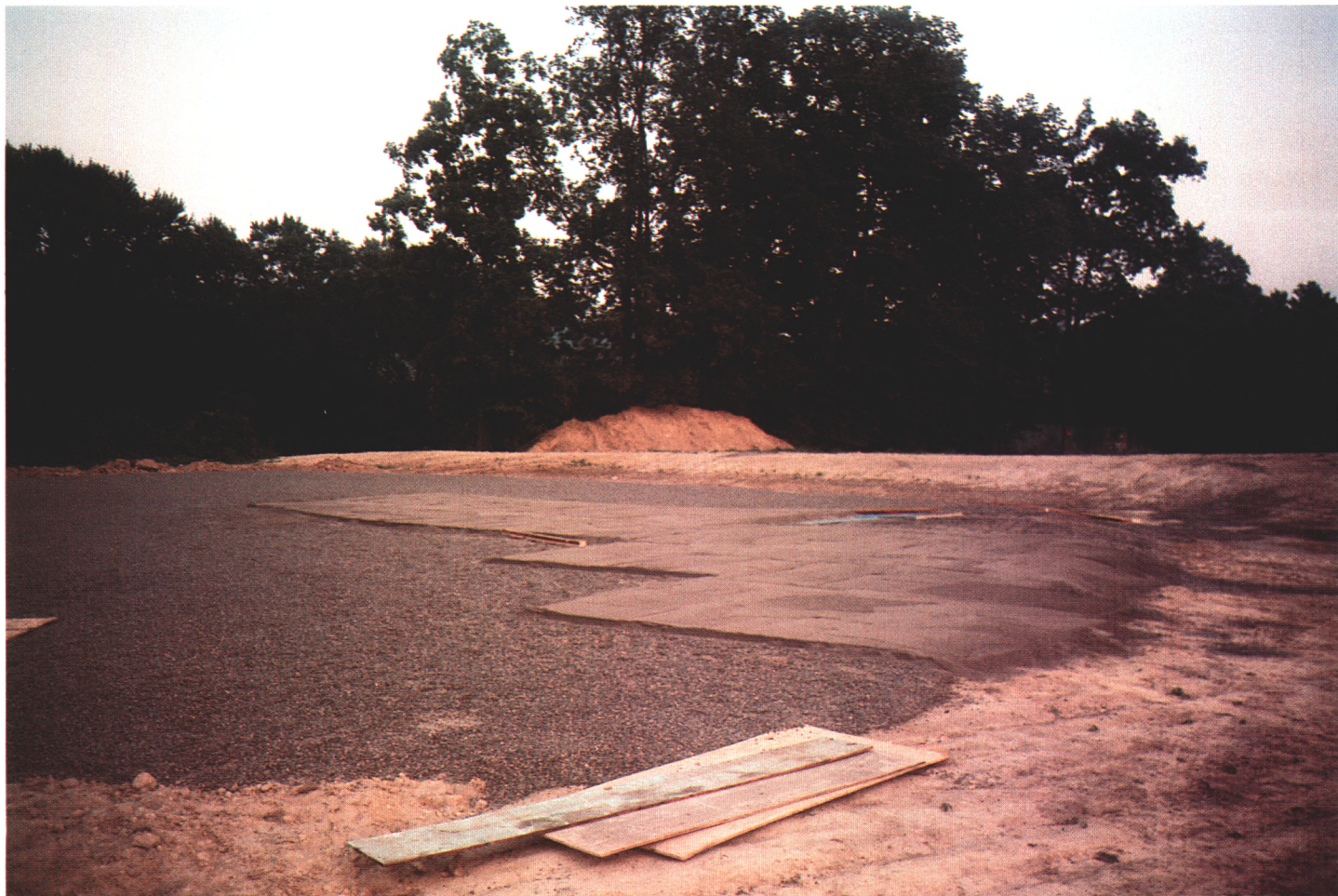
The use of 2" x 4" planks proved most effective for installing a uniform intermediate layer on the new 15th green.
