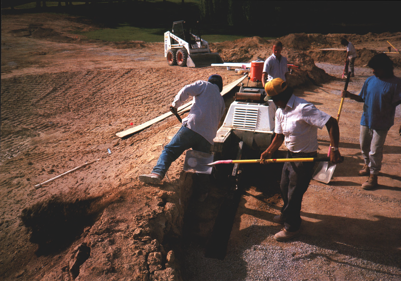
Installation of the "smile" interceptor trench and drain at the low end of a green.
