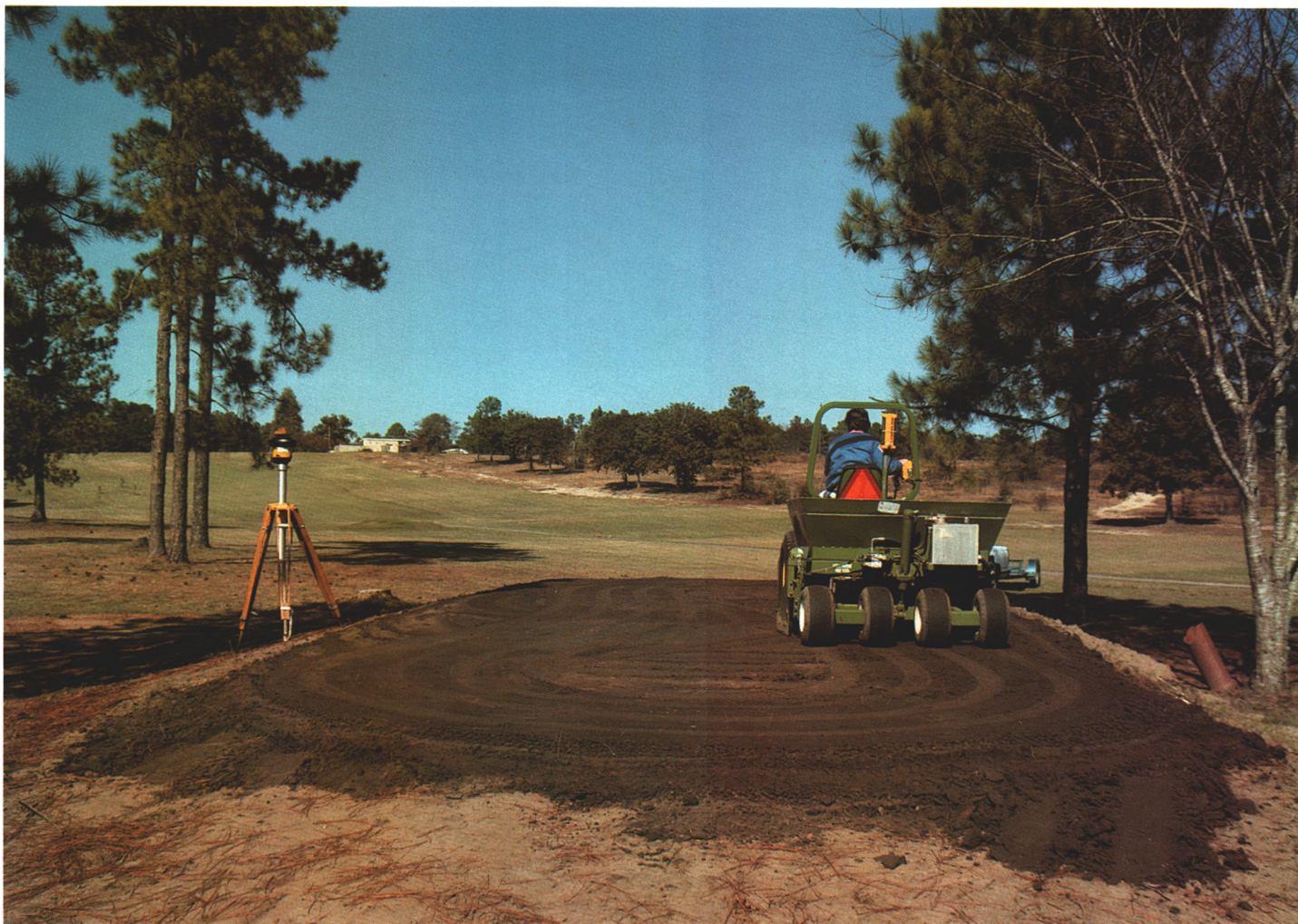
New technological methods have made leveling a tee surface faster and more reliable. Reconstructing tees by a laser-guided grader produces an accurate final product.
