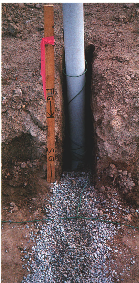
An insulated copper wire, wrapped around the main line, can be used in the future to locate the drainage lines.
