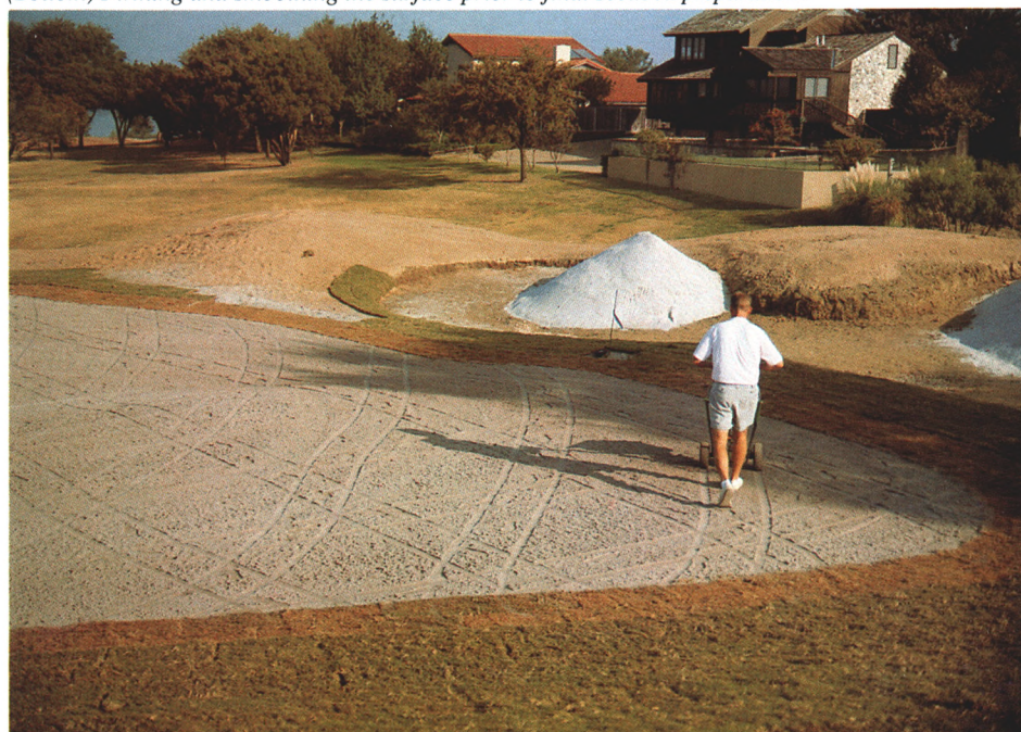
(Below) Almost finished — sowing the seed on a new USGA-standard green. (Bottom) Firming and smoothing the surface prior to final seedbed preparation.
