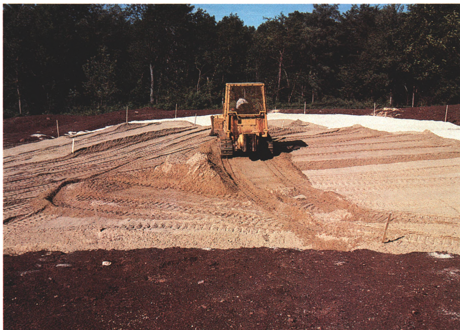
A dozer carefully spreads root zone mix to a depth of 12 inches.
