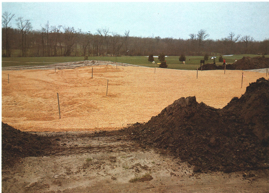
The gravel drainage blanket being laid to the depth indicated on the grade stakes.
