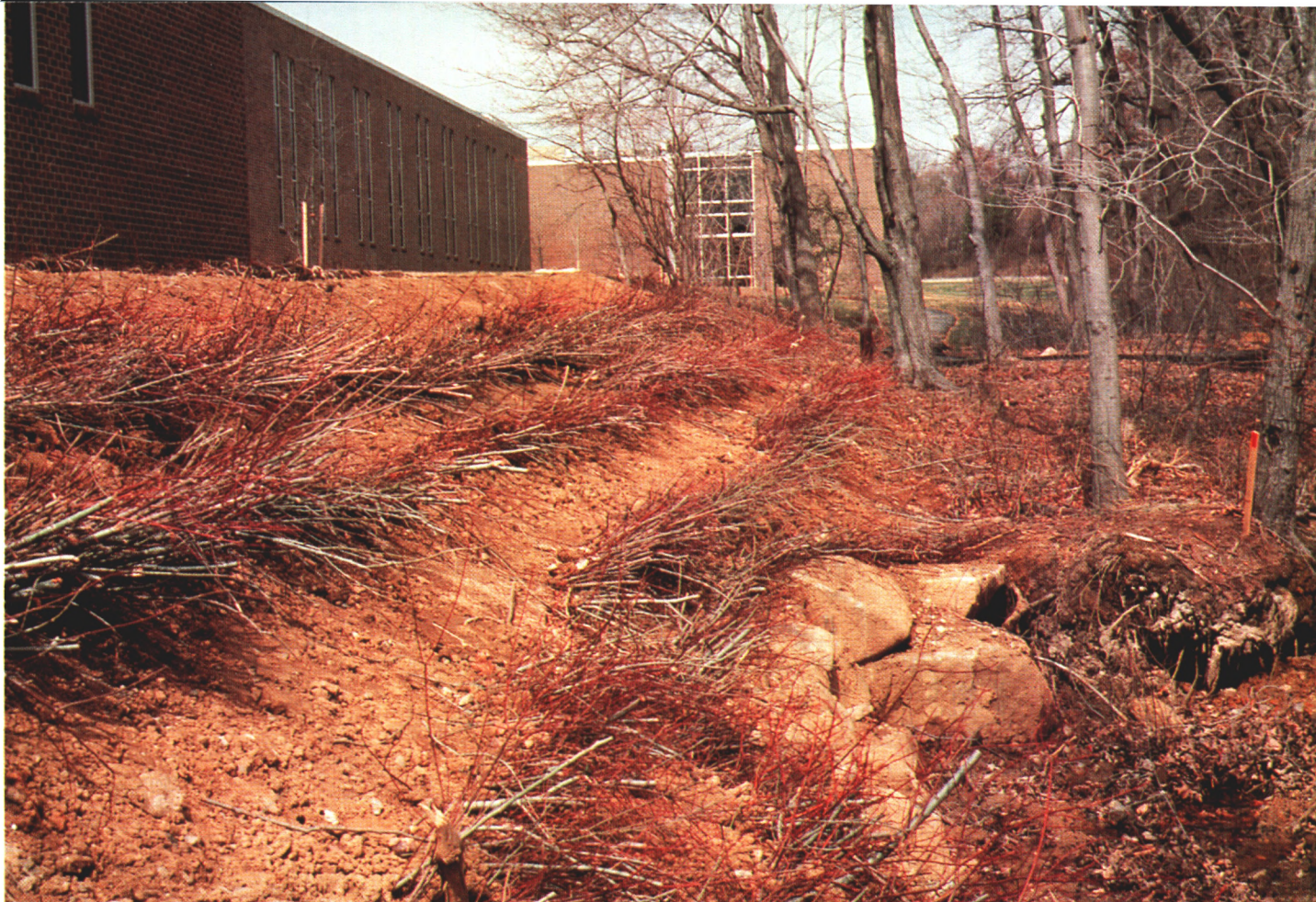
Live willow stakes can be utilized to correct erosion situations. Use of live woody plant cuttings to stabilize severe erosion problems is referred to as "bioengineering."
