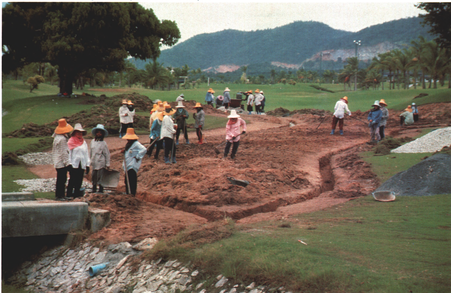
Drainage installation occurring 18 months after construction. Malaysia.
