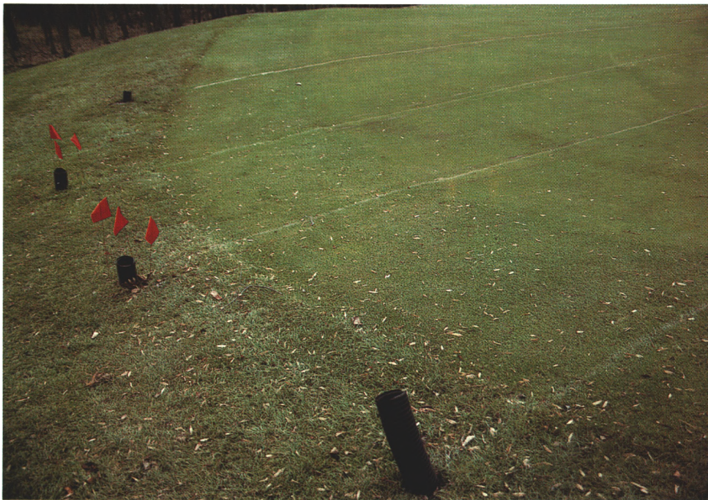
The high ends of the drain lines were brought to the surface, off the green, and eventually were attached to valve boxes for easy access.
