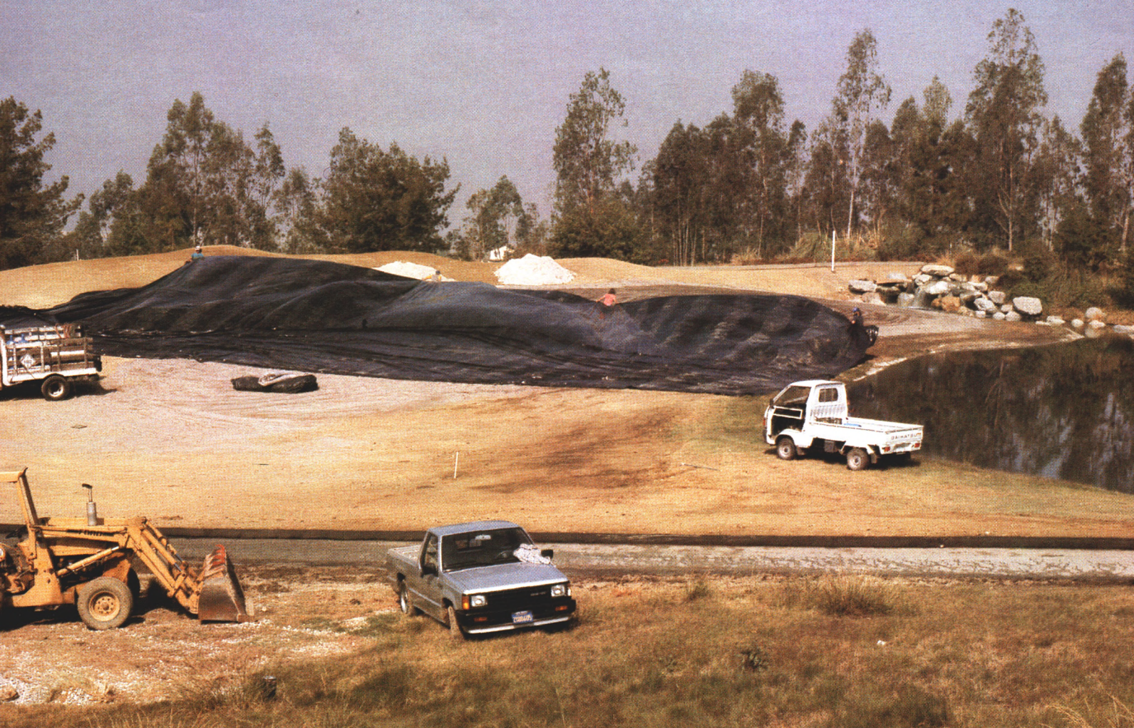
At the Industry Hills Golf Courses, a chlorinated polyethylene liner was installed beneath a methane-affected green to prevent gas migration into the root zone.
