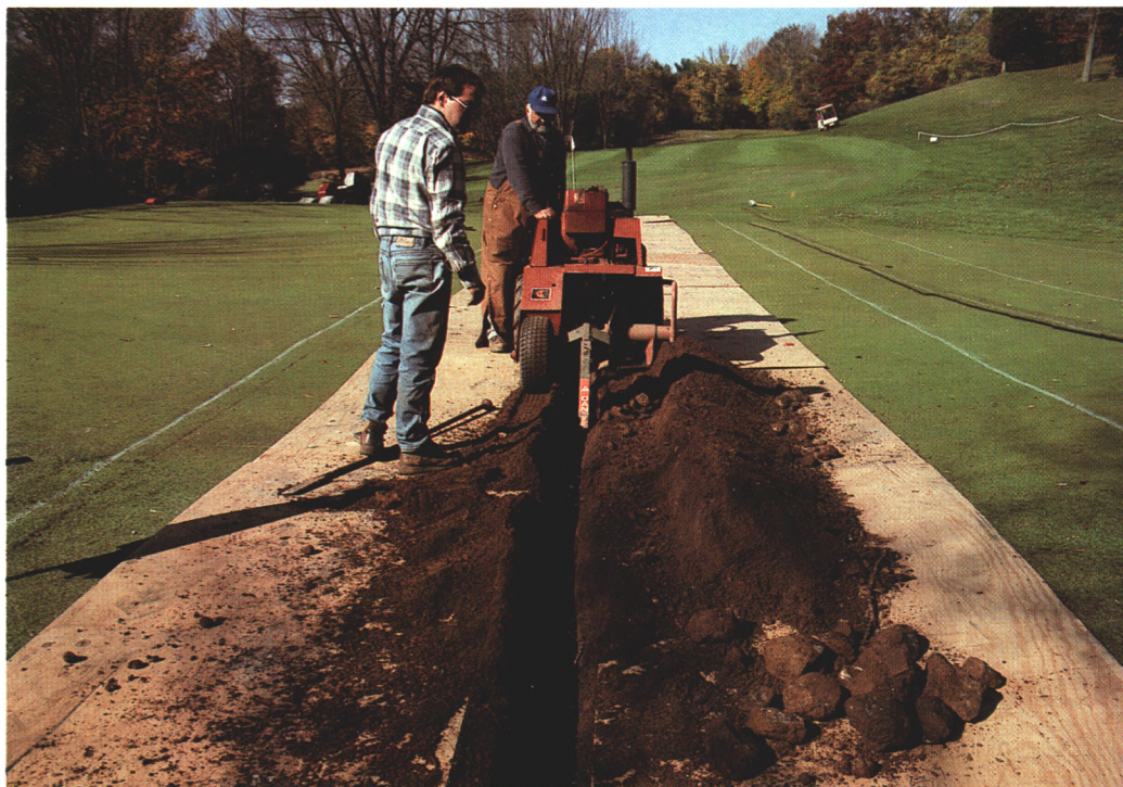
Plywood sheets were laid down along the trench line to protect the turf and make cleanup easy.
