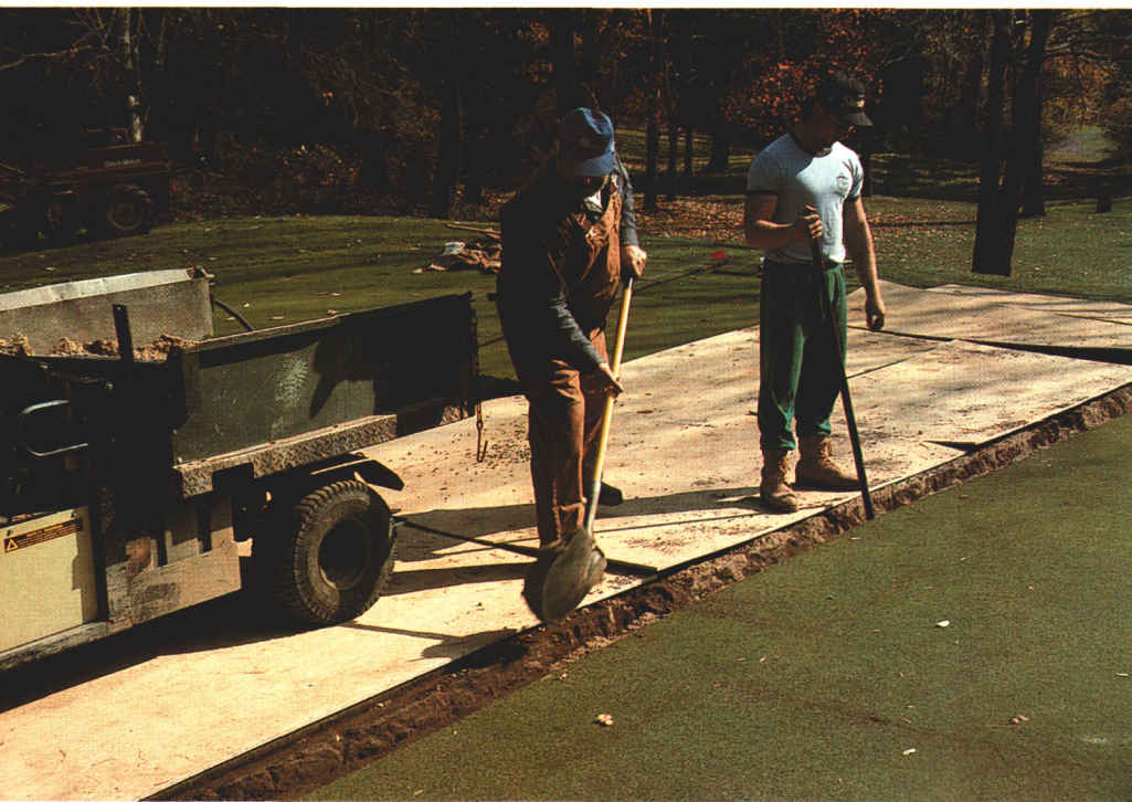
A thin layer of gravel was put in the trench, followed by 3-inch perforated drainage tile and more gravel. Topmix was added and tamped in layers to minimize possible settling problems.
