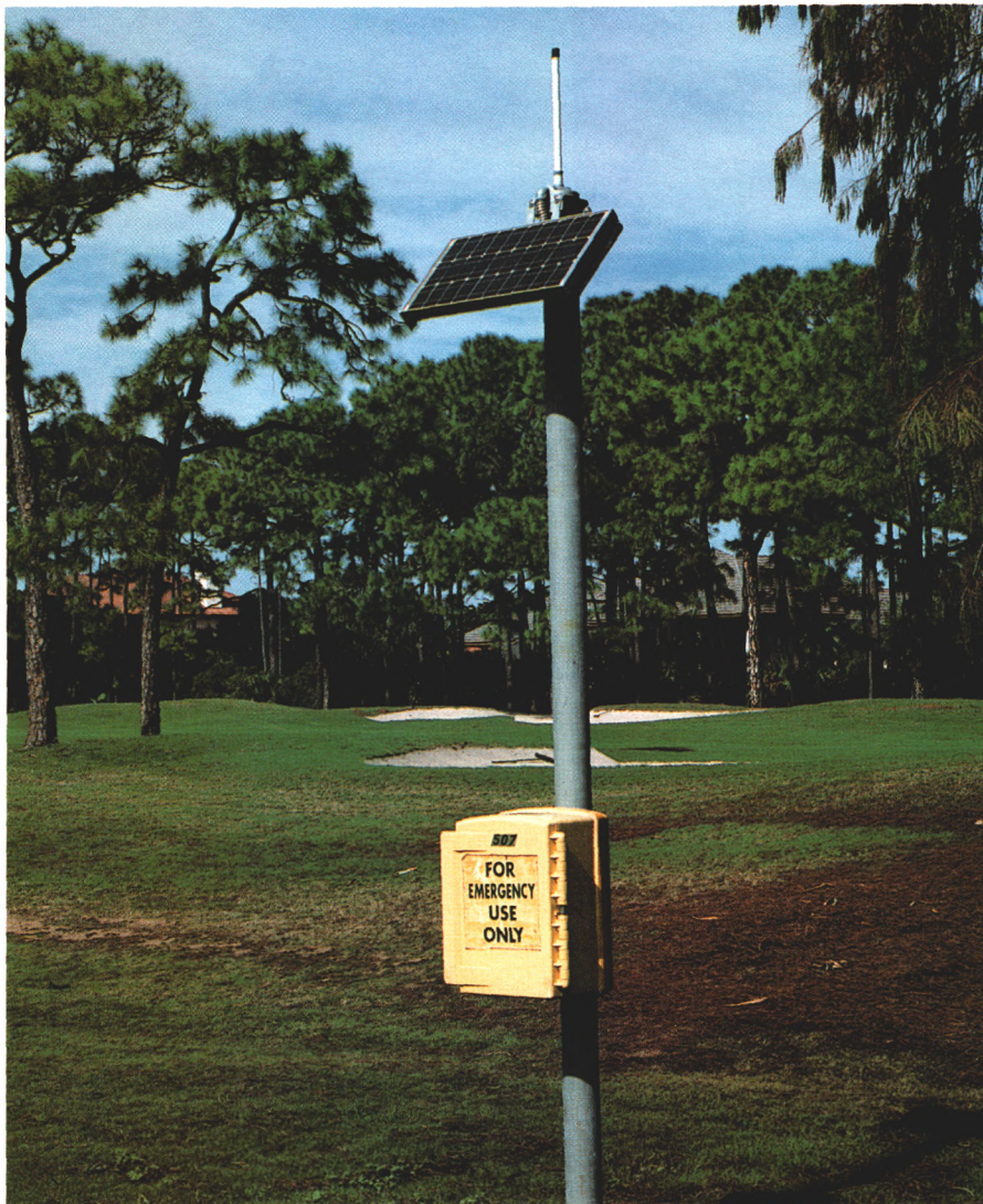
The installation of emergency call box systems on golf courses has been streamlined through the use of wireless communications equipment.
