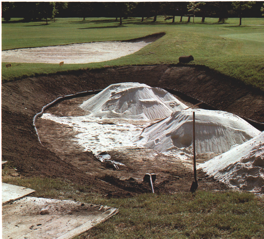
During the Acacia Country Club bunker renovation, drainage pipe was used to delineate the renovated bunker edge.
