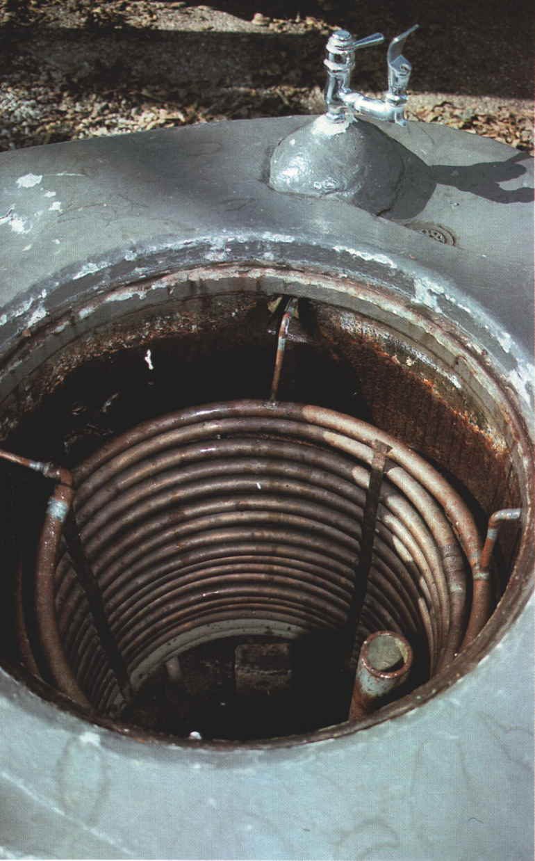
A continuous coil of 1" copper tubing brings water from the supply to the fountains.
