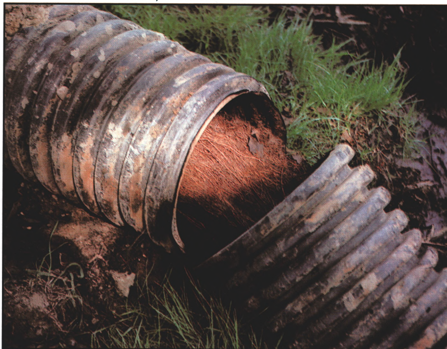
This 12-inch drainage pipe was filled with willow roots three months after installation.
