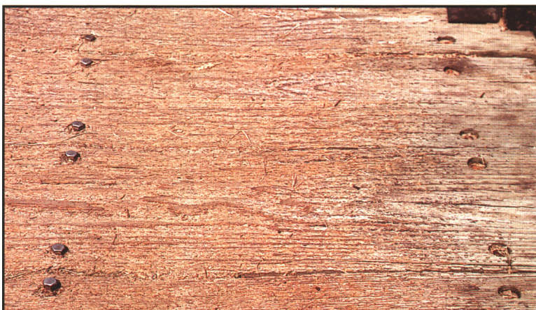
Metal spikes can cause significant damage to non-turf areas. The counter-sunk bolts on this bridge have been exposed as metal spikes have worn away the wood on the trafficked portion of the bridge.
