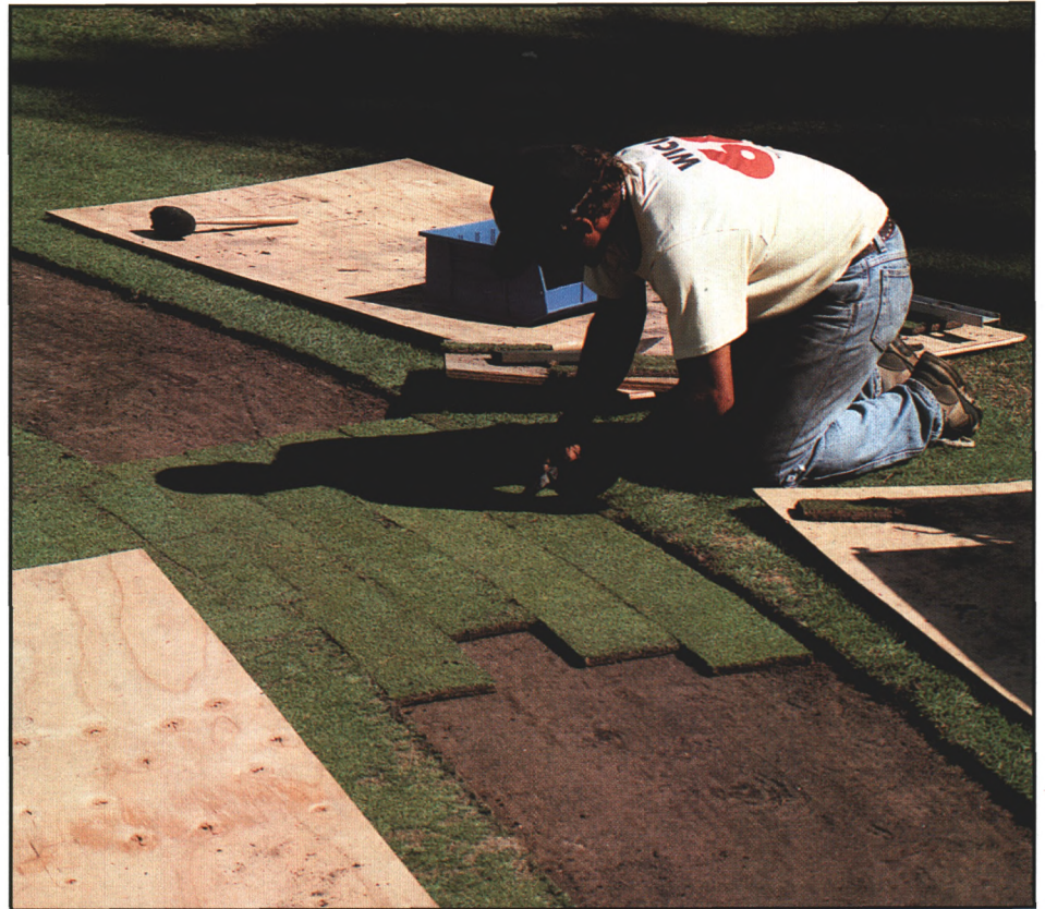
Nursery sod is carefully installed after underlying soils have been graded and rolled.
