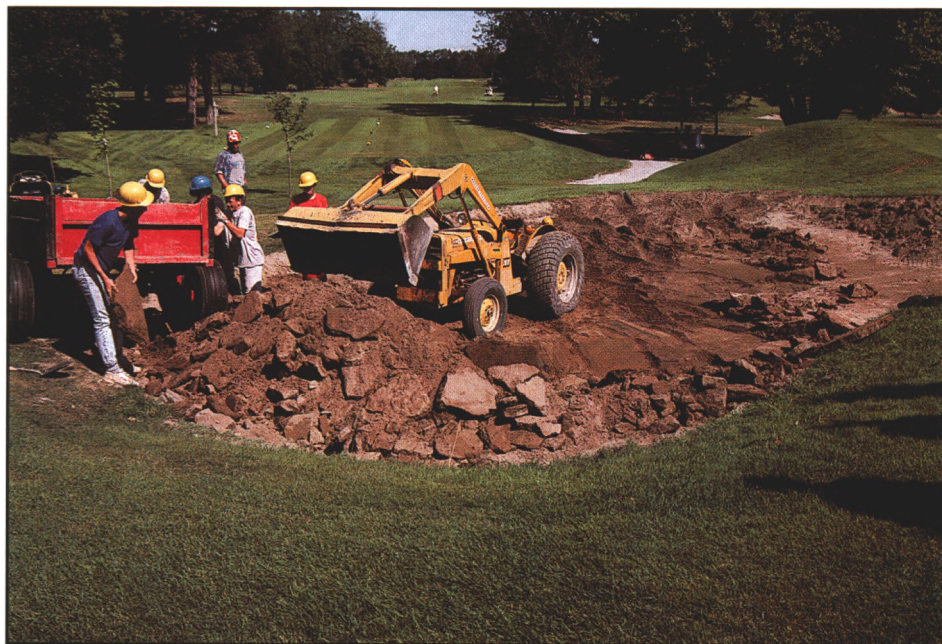
Proper sand selection is one of four components in evaluating bunker sands. An improper choice at this course resulted in cement-like slabs that required complete removal soon after installation.
