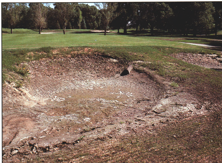
Thick layers of silt and other debris contaminated the bunkers throughout the golf course. In many areas, swift currents washed the sand completely from the bunkers. Complete renovation was necessary on several holes.
