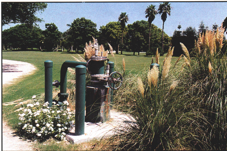
A 1,500-foot-deep artesian well supplies brackish water to the reverse osmosis plant at the Jupiter Island Club (Jupiter, Florida).
