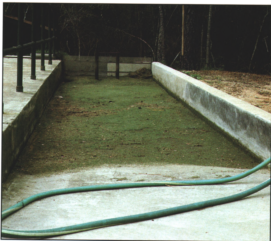
A unique wash area and rinse system was implemented at Pinehurst Course #8 to retain all water on-site. The system uses a series of natural filters to cleanse wash-down water before it is discharged onto the turfgrass.
