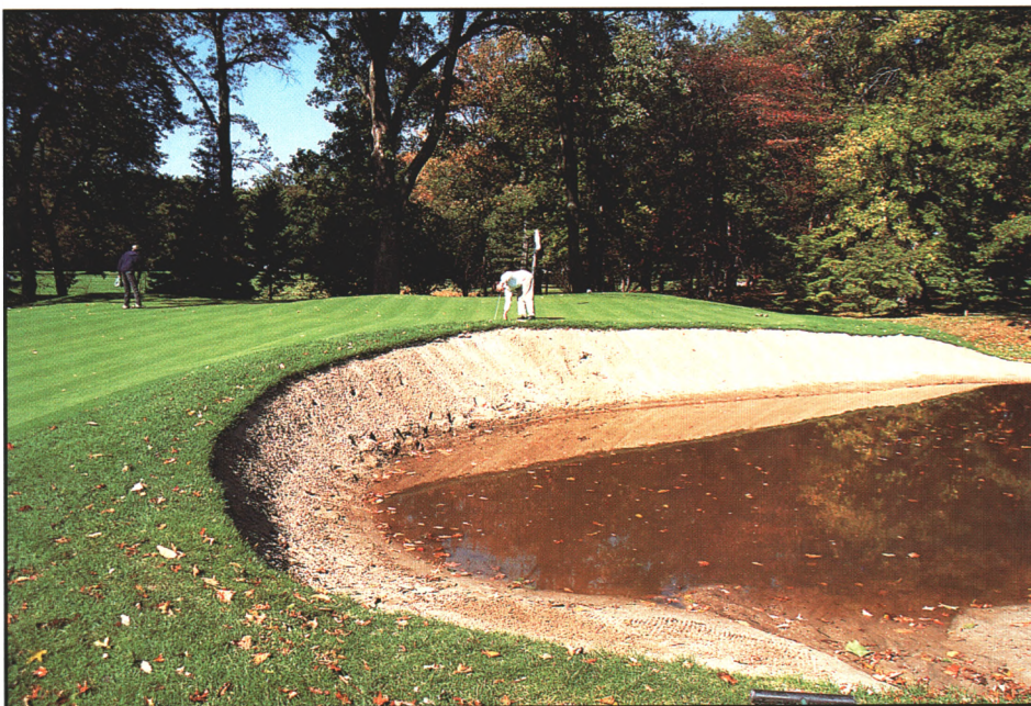
At times, water accumulates in a bunker faster than the subsoil can absorb it. In sandy soils, no drainage system may be necessary, but in clay soils a properly functioning drainage system is a must.
