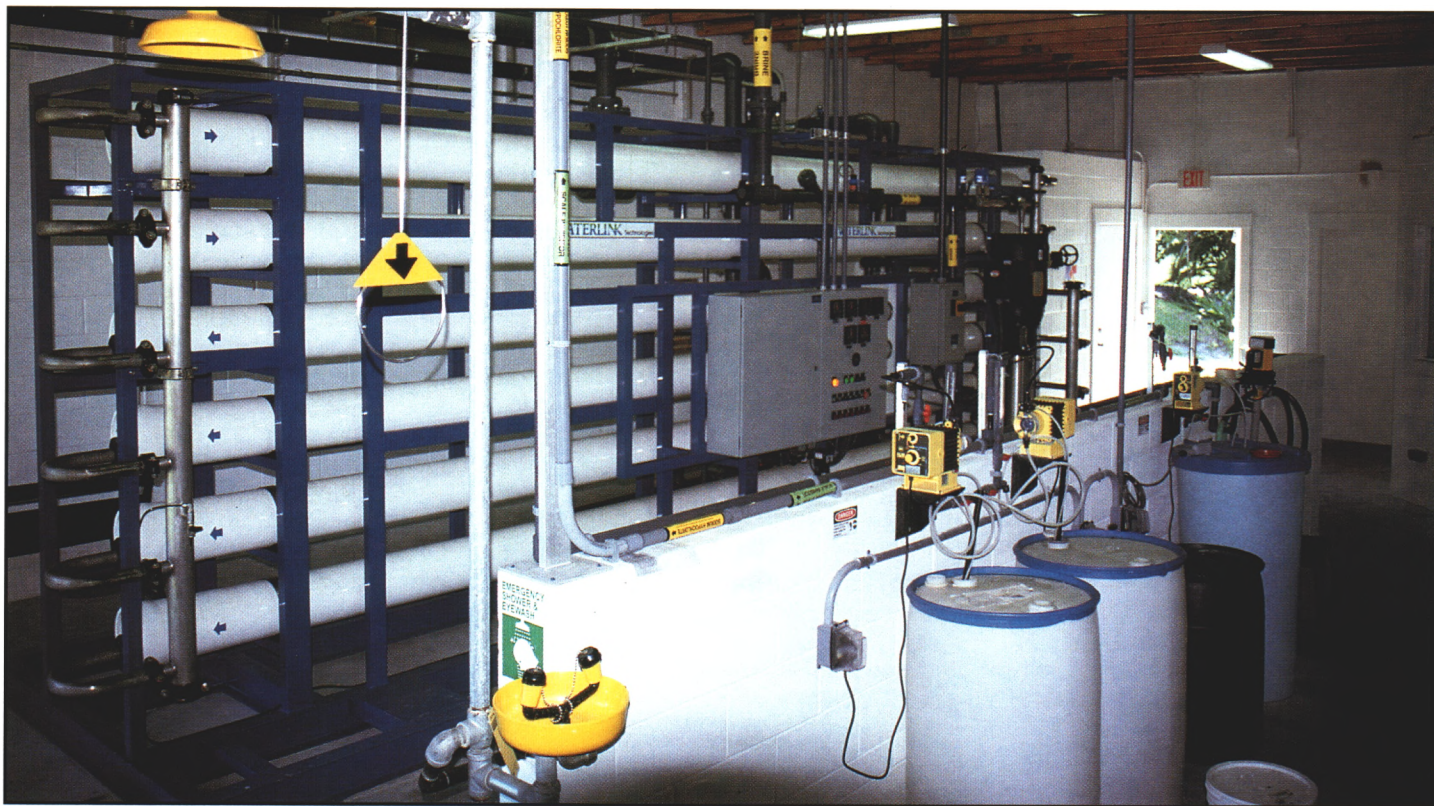
The filtration vessels are at the heart of the reverse osmosis water treatment process. For every four gallons of brackish water treated, three gallons of usable water is produced.
