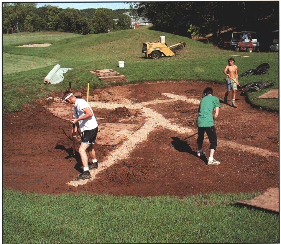
Proper internal drainage is a must for a bunker to be successful in the long run.
