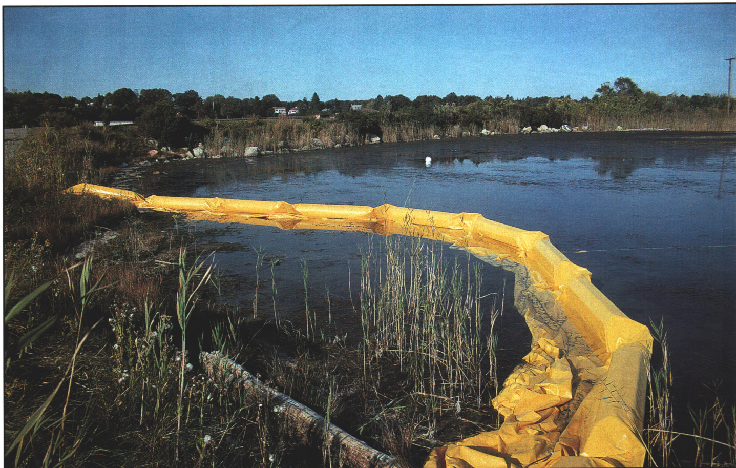
A containment device is used to protect wetland areas from siltation caused by nearby construction work.
