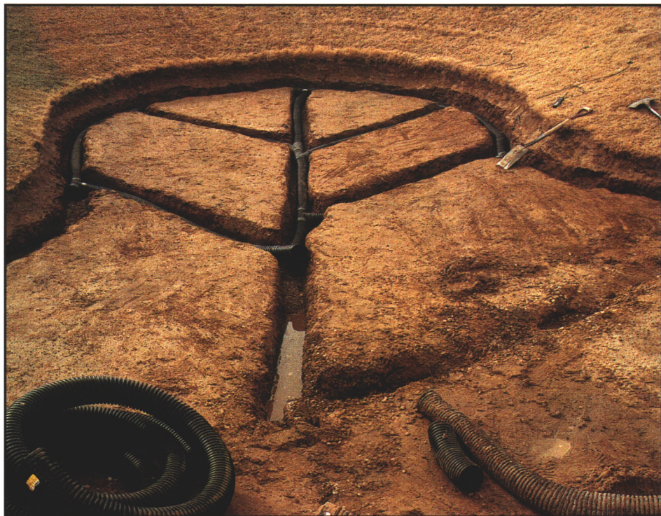
Installing a perimeter drain line under the edge of steep bunker faces can prevent erosion. During a heavy rain the extra drain line captures water from surrounding turf areas and prevents the sand from becoming saturated.
