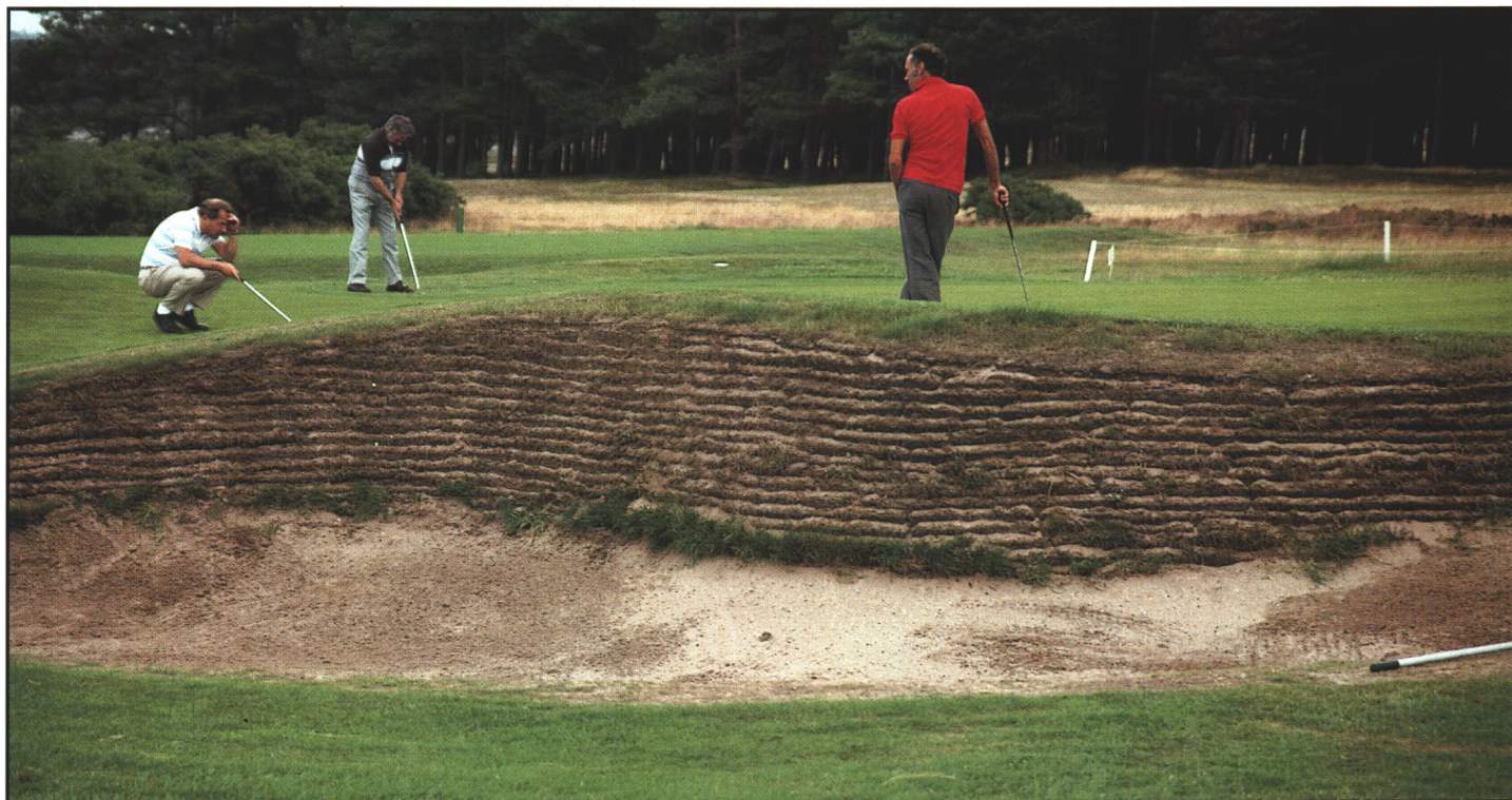
Revetted bunker faces are constructed by stacking thick pieces of sod. The life expectancy of turfed bunker faces depends greatly on orientation to the sun.
