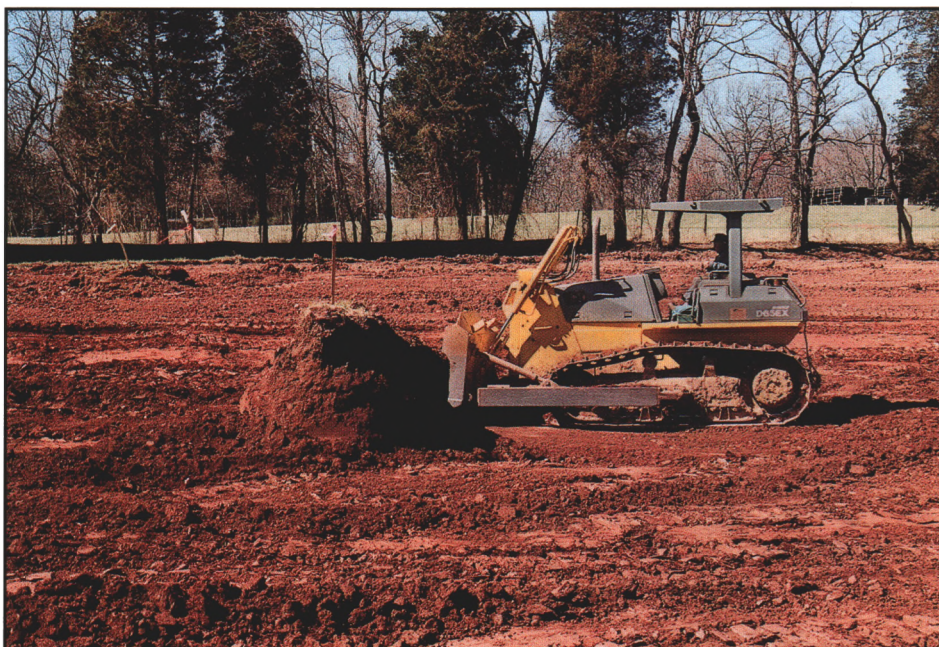
Heavy earth moving is expensive. This operator is making a cut of at least five feet.
