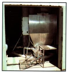
Acid injection and sulfur burners can be used to treat water with excess bicarbonate levels. Acidifying irrigation water to a pH of 6.5 reduces bicarbonates by approximately 50%.
