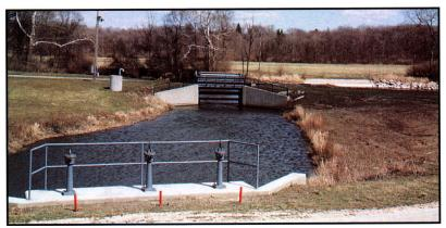
A selfcleaning screen at the lake intake prevents large debris from entering the system.
