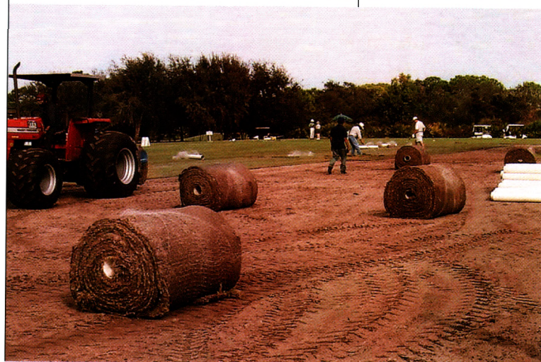
Thick cut, big roll bermudagrass sod is used to re-grass the back half of the practice tee. Rolling out the carpet on the practice tee has proven to be the best option for accommodating the golfers.
