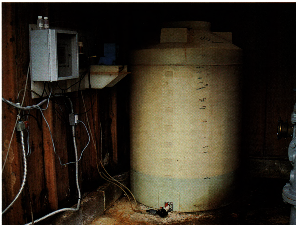
The direct injection of sulfuric acid into the irrigation mainline from a nearby storage tank is another method to introduce acidifying amendments. The hazard of handling concentrated acid must be considered along with the need to provide adequate space at the pump station for the storage tank and access by delivery trucks.
