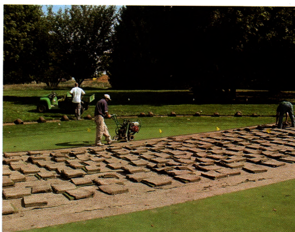
To begin the recontouring project, Baltimore Country Club (Maryland) stripped and folded the sod prior to removing it from the 12th green.
