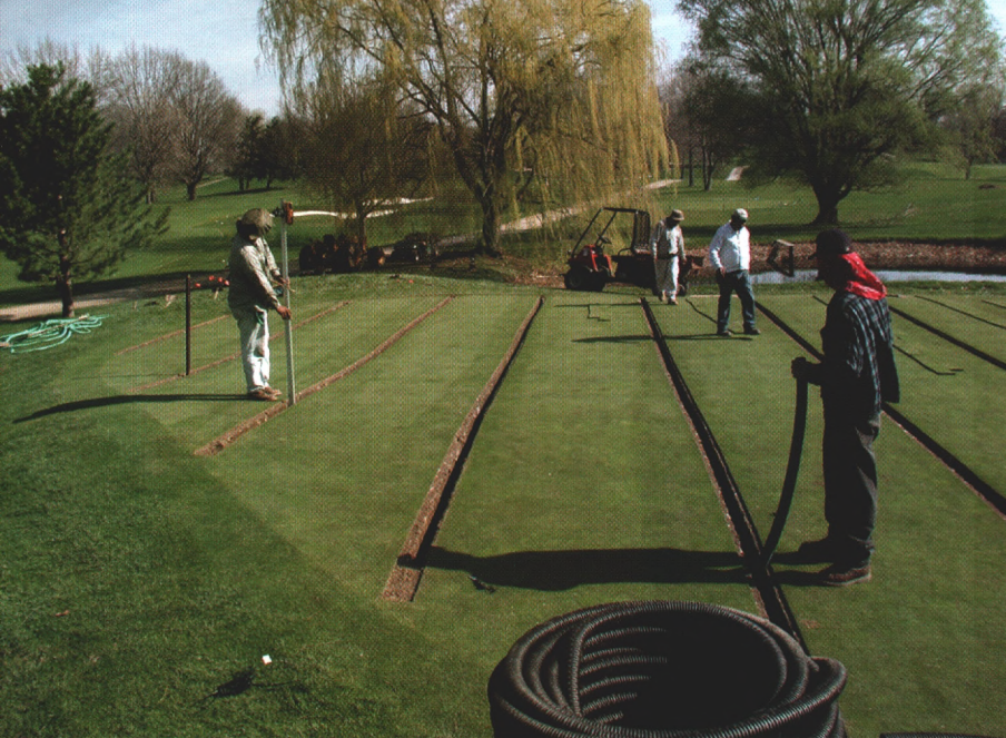
Subsurface drainage installation is tedious work that is often best left to the expertise of a drainage contractor.
