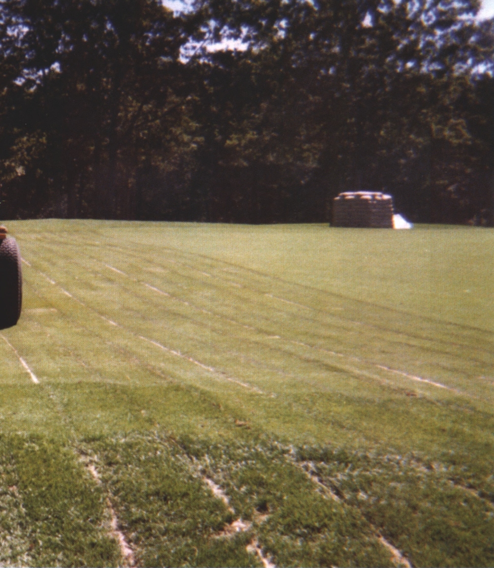
Installation of slit drainage is effective, but it is usually more disruptive than subsurface drainage.
