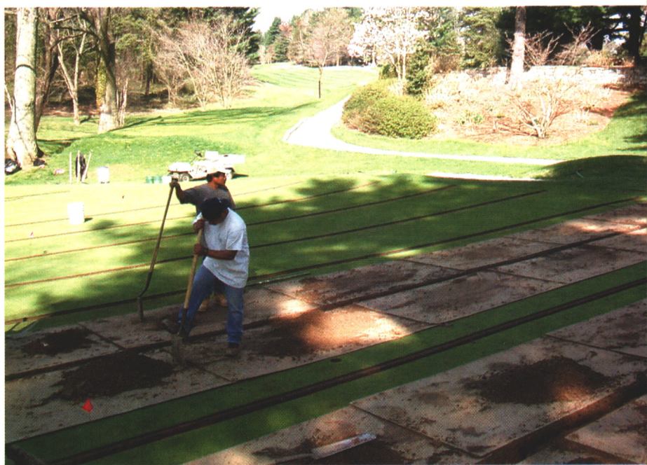
Installation of internal drainage in older, soil-based greens greatly improves their chances for survival in general, but especially under poor weather conditions with wet patterns and high temperatures.
