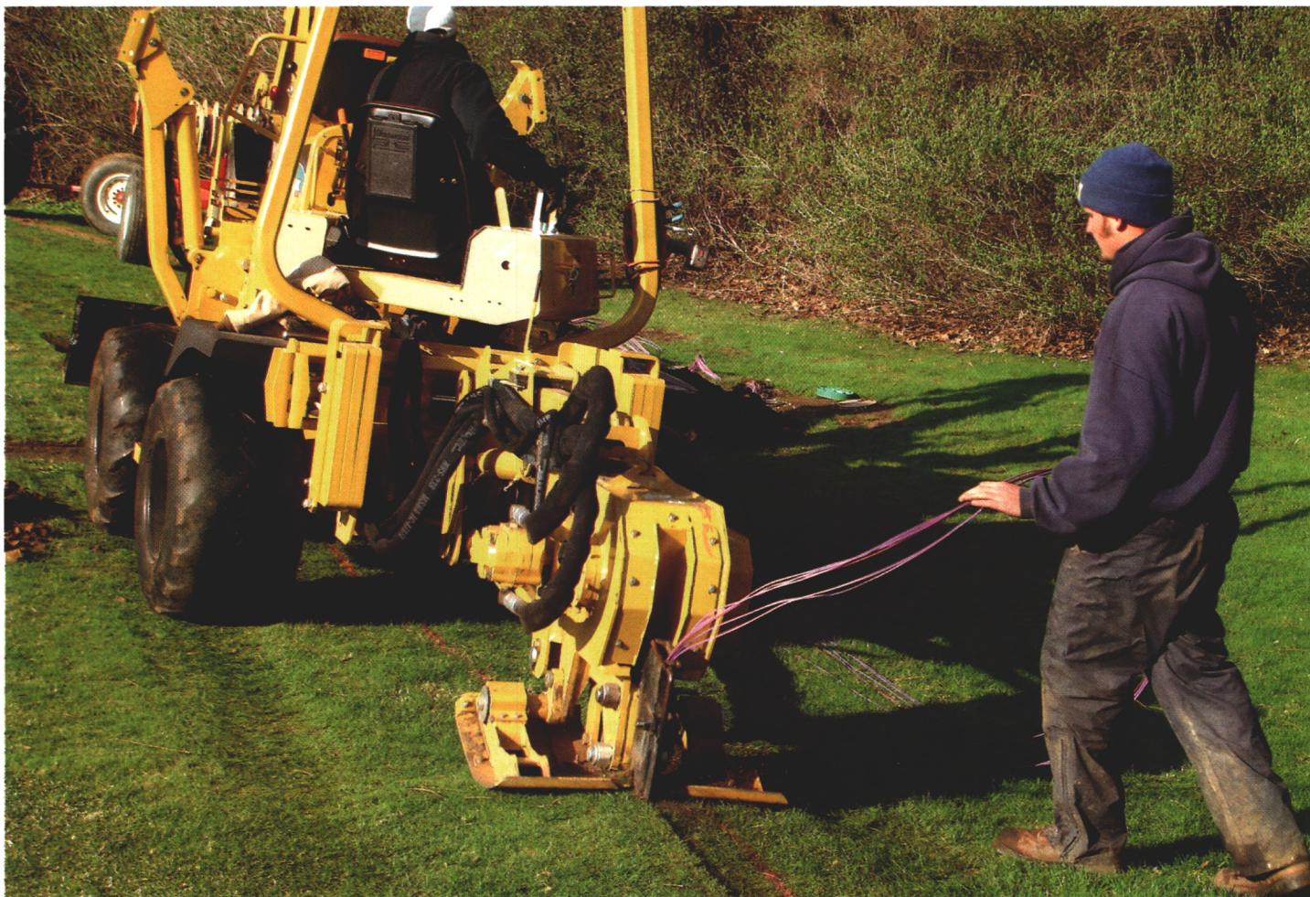
Wire should be laid, not pulled directly off the roll.
