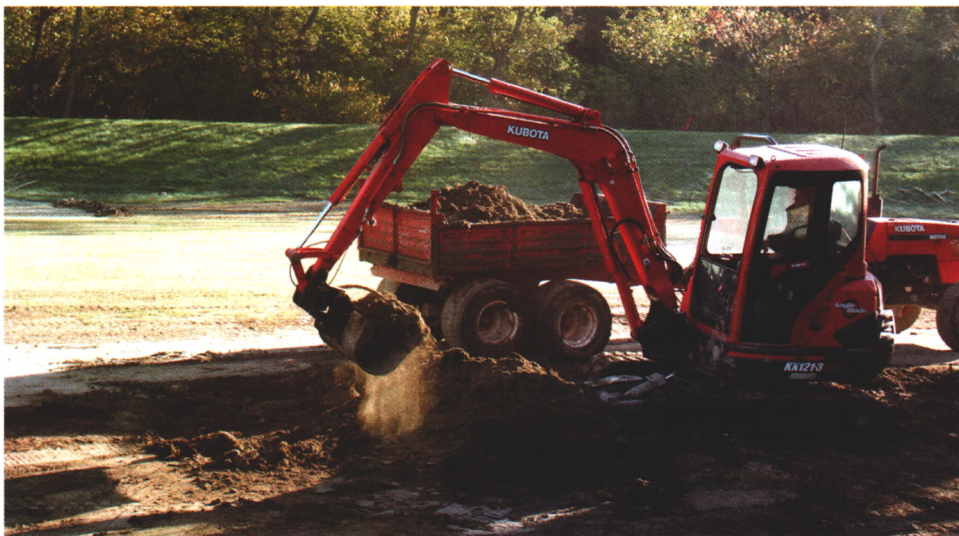
We employed the services of an outside contractor to remove severely contaminated bunker sand. Unfortunately, the damage occurred only a few months after we had completed a major renovation of all of the bunkers.
