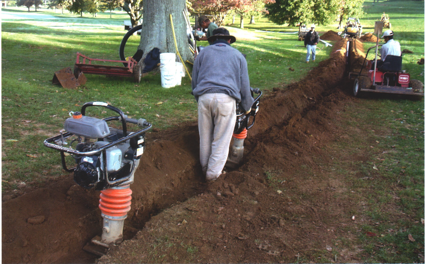
Proper compaction, in lifts, with mechanical equipment is an important consideration in the installation process.
