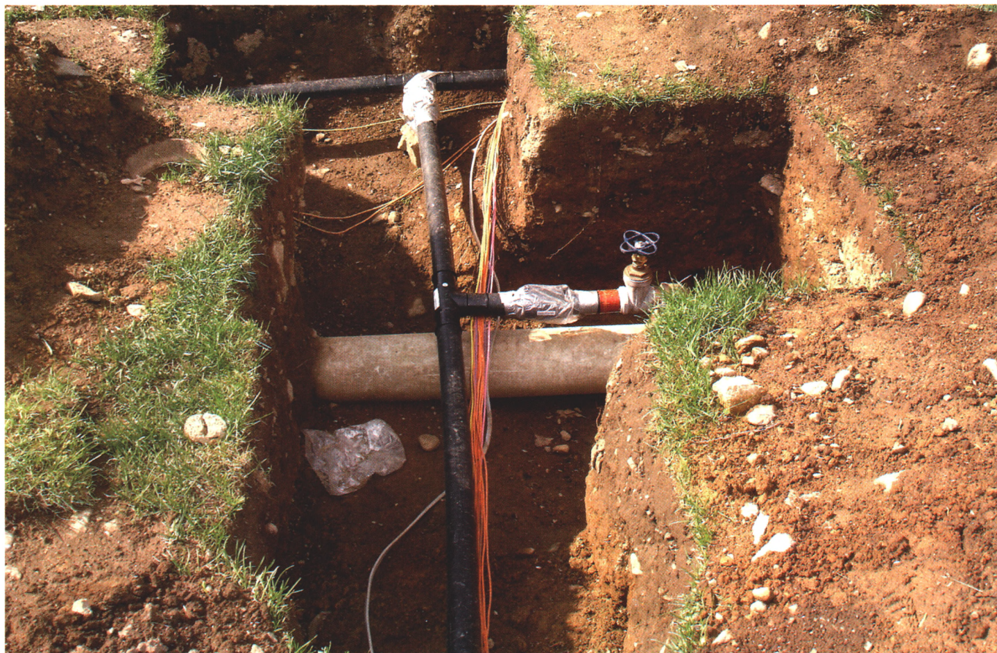
Proper pipe burial depth should be maintained throughout the entire irrigation system installation.
