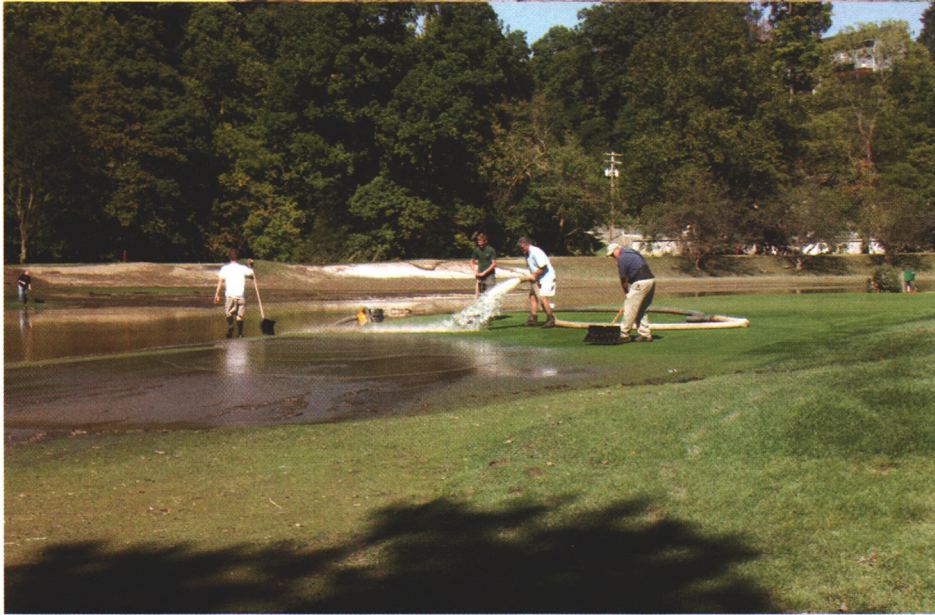
Large trash pumps moved high volumes of water over silted areas of the golf course. Once a slurry was created, it was moved with plastic snow shovels.
