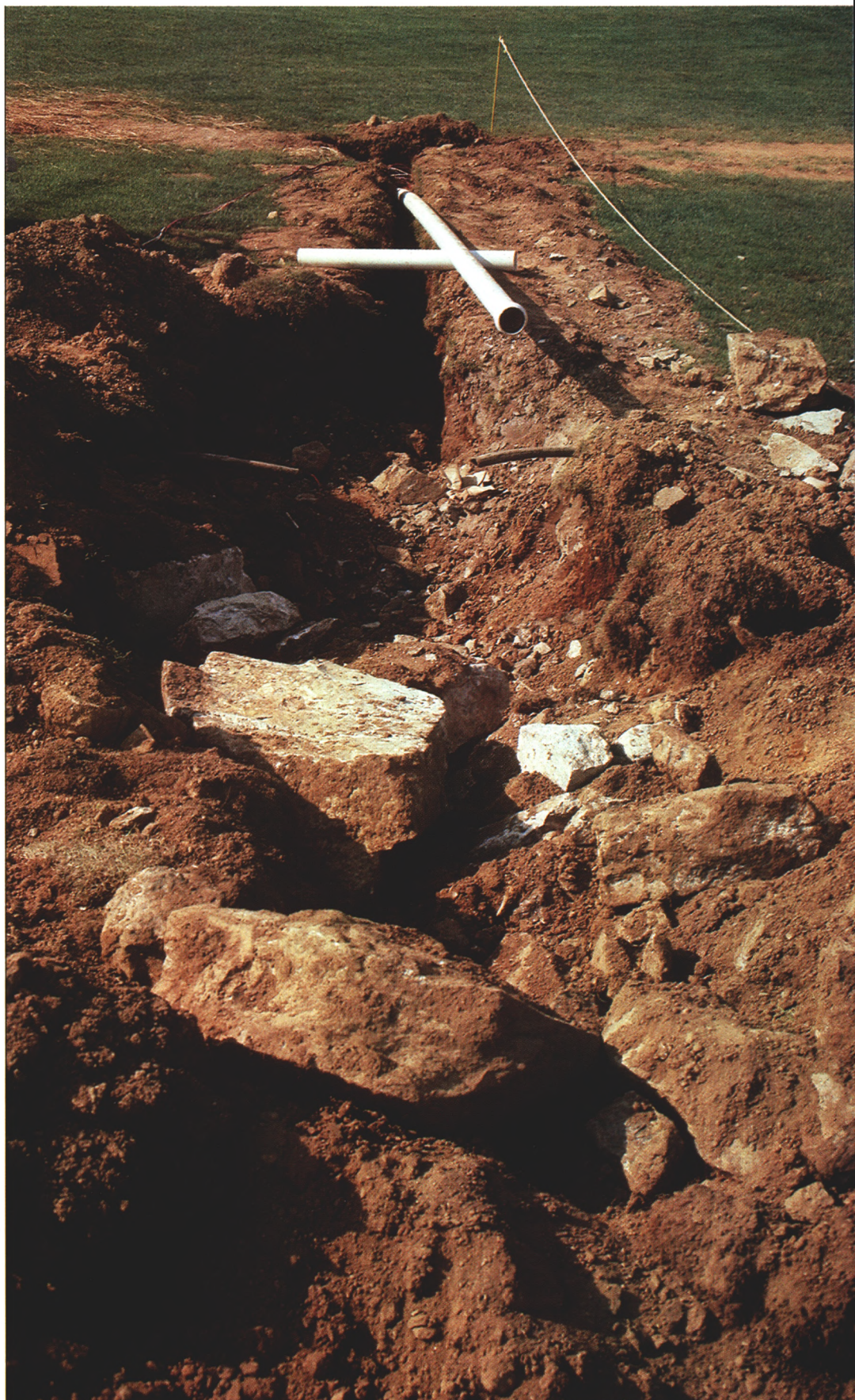
Rock can add significantly to the irrigation system installation cost. These conditions need to be carefully budgeted.
