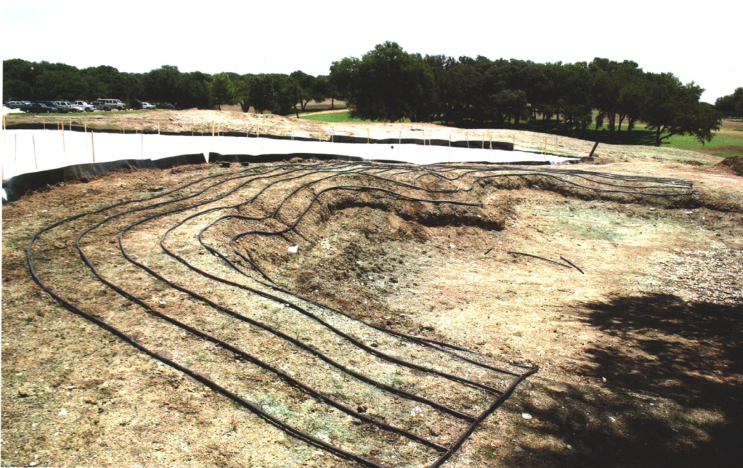
A subsurface drip irrigation system was installed in the grass face of the bunker adjacent to the experimental green. This allows the turf on the face to be irrigated without overwatering the adjacent areas.
