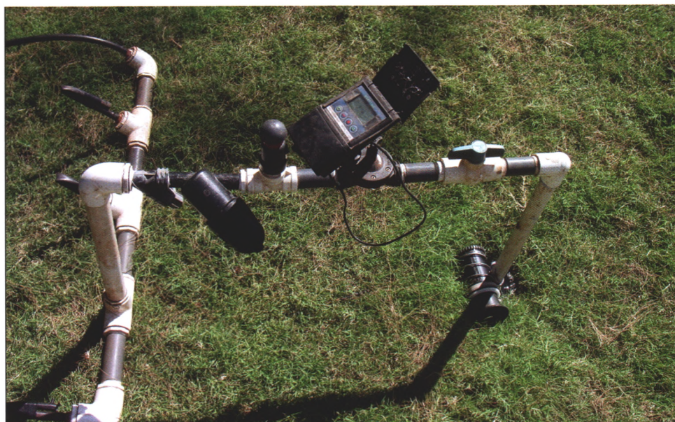
The Turtle Bay Golf misting system is adapted to larger sites with multiple lines sent from the control system. The lines have been pressure reduced from the regular irrigation system.
