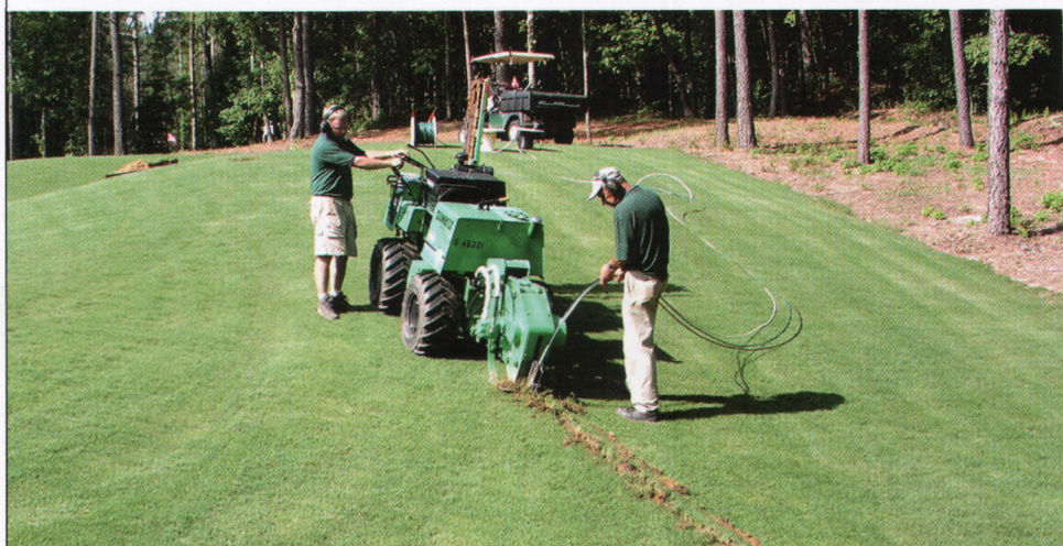
Wire materials and installation are the most expensive costs for a fan project. Installing the wire to the proper depth and according to local electrical codes is essential to supply consistent power to fans.
