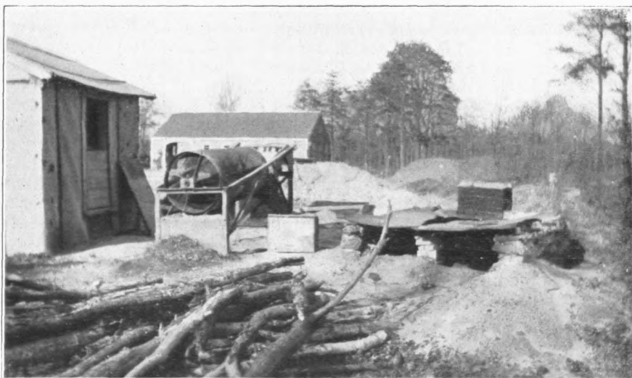
Soil-baking oven for killing weed seeds.
