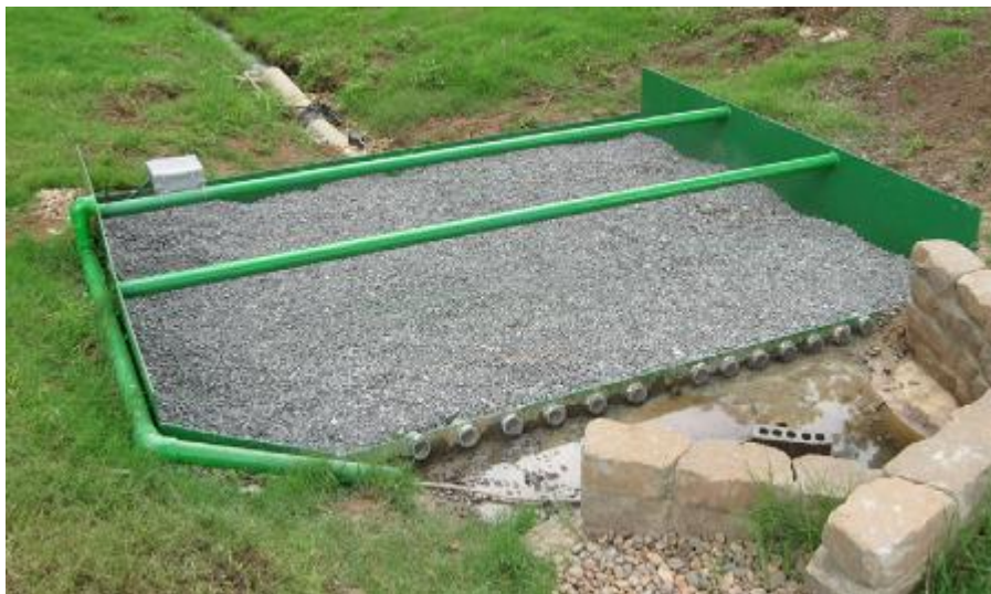
The completed phosphorus removal structure filled with steel slag, a byproduct of the steel production industry.
