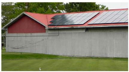
Solar panels were mounted atop roofs of the maintenance facility, pool house, and cart barn to limit their aesthetic impact. The savings in electricity costs combined with the sale of SRECs (Solar Renewable Energy Credits) back to the power grid will recover the cost of the investment in less than five years.
