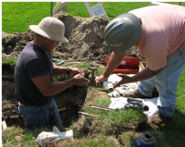
Valve failure and frequent pipe breaks are signs that parts of an irrigation system are worn out and need to be replaced.
