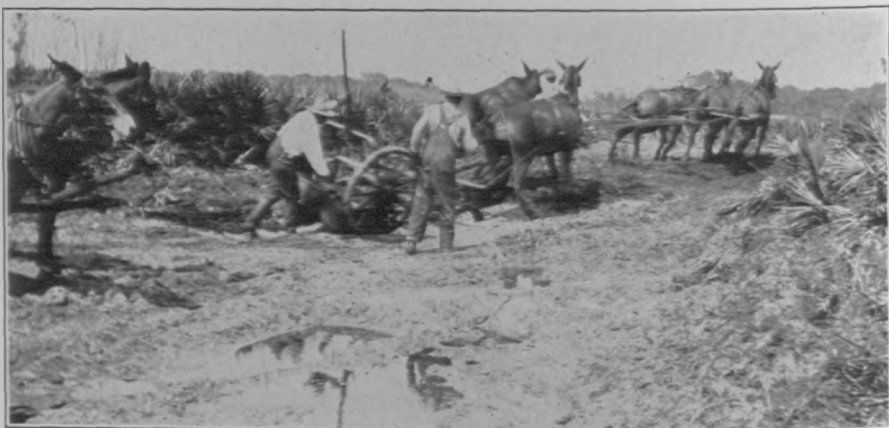
Snatch team loading a wheel scraper.
