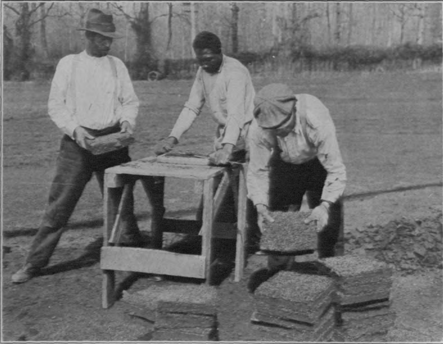
Trimming sod to an even thickness by using a cutting box.
