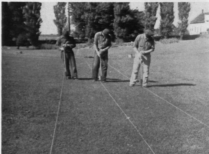
Weed canes for treating scattered weeds. By this method small quantities of chemicals can be applied to individual plants in a clean-up job.
