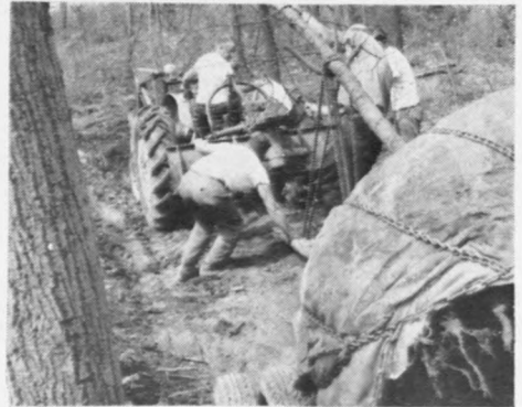
6. By the fulcrum principle, the tree is eased now into a horizontal carrying position.
