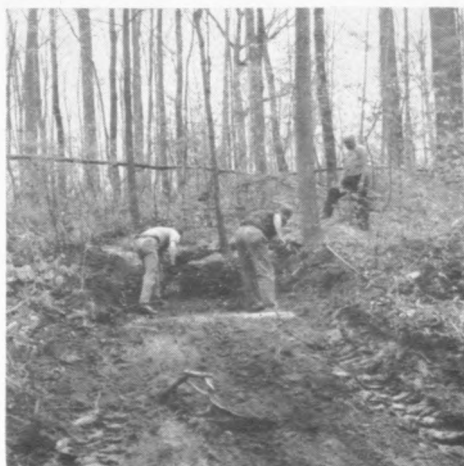
2. The rough digging is done by a front end loader or backhoe. A minimum of fine work with pick and shovel is required. The tree is selected from the wooded area on the course.
