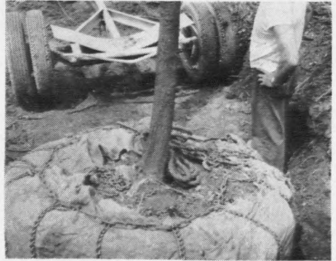
4. The ball is firmly held by burlap and chain and the tree mover is being backed into position.
