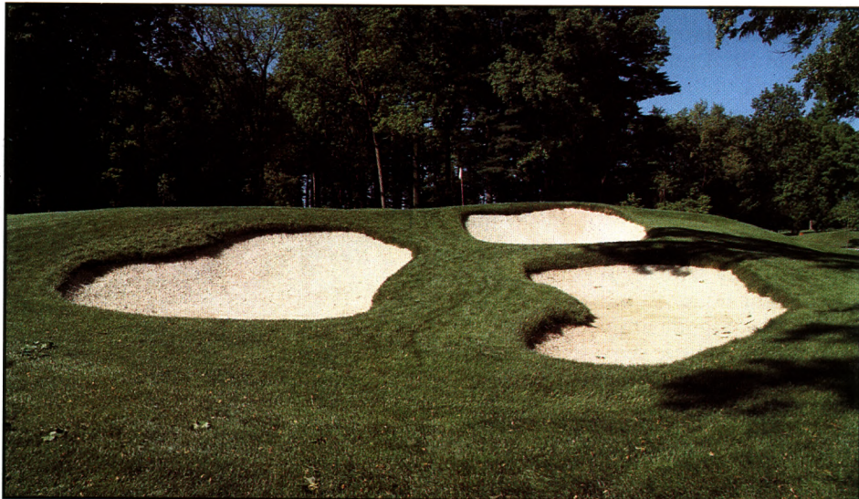
After renovation, the bunkers were slightly larger and deeper with distinct faces as a result of the stacked sod method employed. More importantly, the finished product fit in with the overall character of the golf course.
