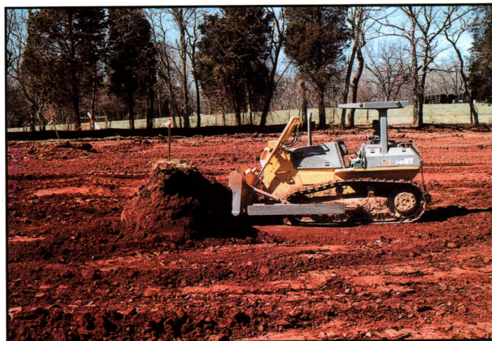
Soil moving is often the most expensive aspect of golf course construction. Deep cuts such as this require the movement of tremendous quantities of soil.
