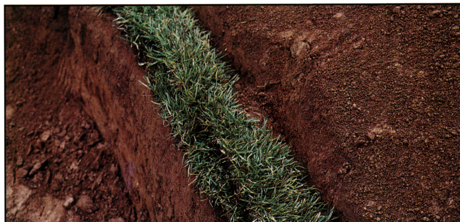
With each layer, soil was added and compacted between the sod and native soil. Tight compaction of the soil behind the sod was imperative to prevent the sod from shifting.
