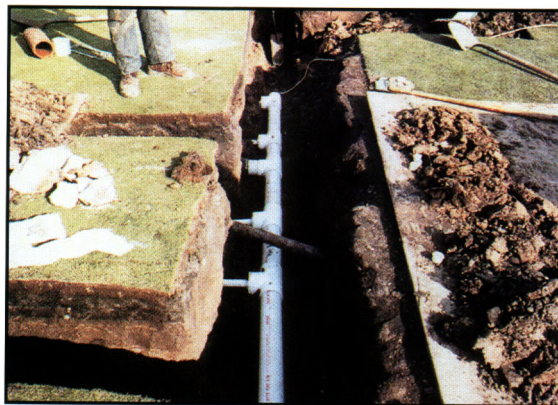
After several lateral drain pipes have been pulled underneath the ground by a boring machine, they must be connected to a mainline that allows excess moisture to escape from the green. Connecting the drain pipe to a main line requires digging a narrow trench off to the side of the green, where the disruption will have little impact on play.
