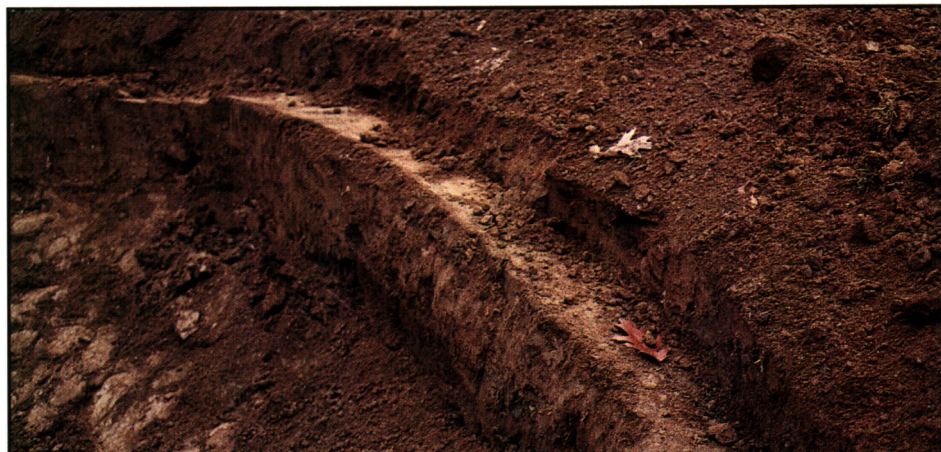
A soil ledge approximately 10 inches in width was created to provide the initial footer to begin stacking sod.
