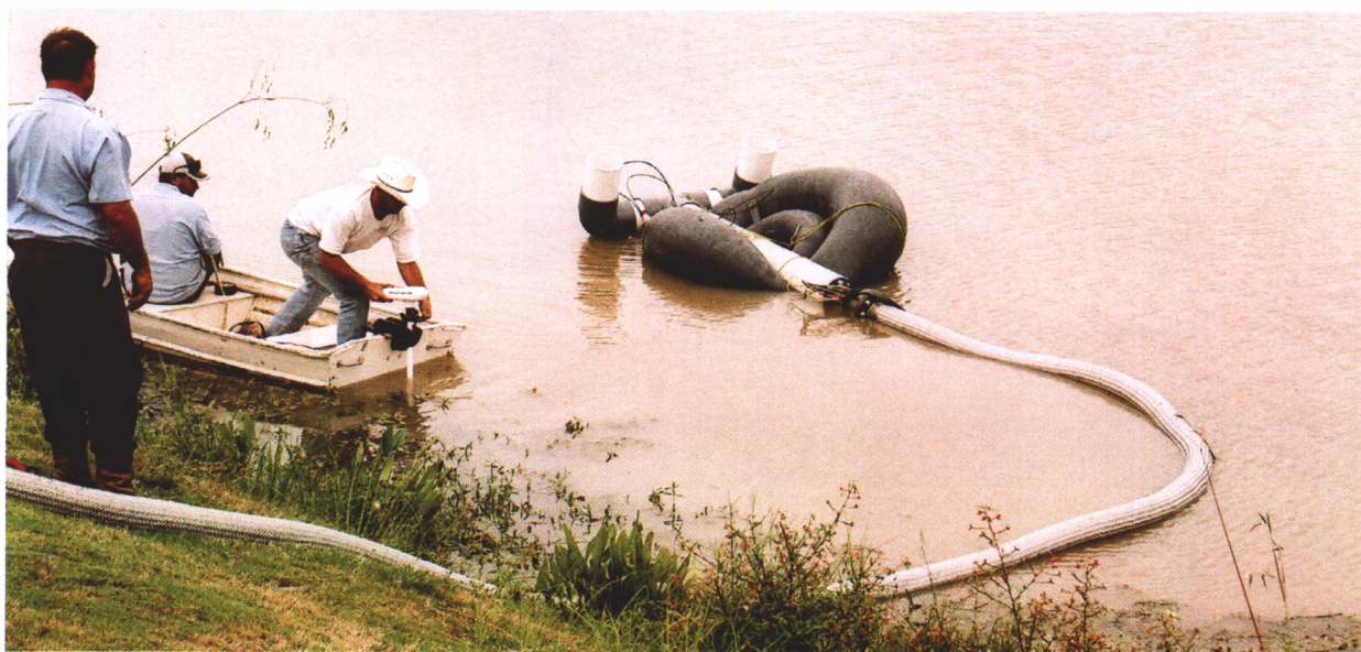
This photo shows the installation of a submersible diversion pump so another structure is not seen on the golf course. The maintenance of submersible pumps is not difficult.
