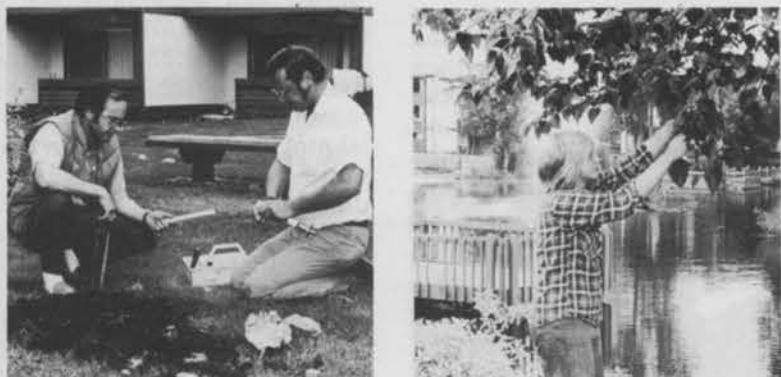
Owner Mike Jones (left) and foreman Harold Caruthers repair a sprinkler system. Once Jones got good workers, he was able to instill in them a pride for their work.
