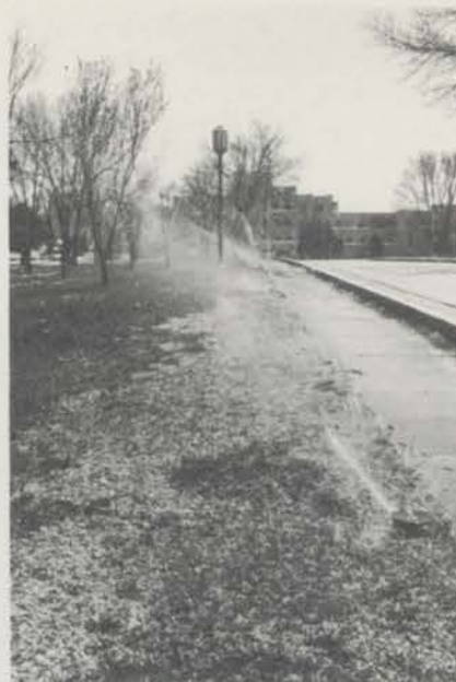
Nearly 1,000 sprinklers were utilized in the irrigation system installed on the 85-acre VA hospital complex in Albuquerque, N.M. Some of the facts and figures on how money was saved by installing an automatic irrigation system might be useful to a lawn care businessman on his next irrigation sale.
