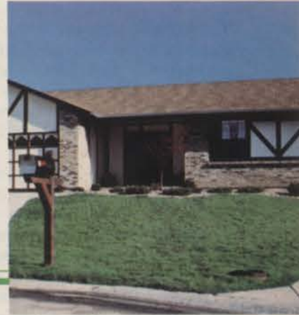
5. COMPLETED RENOVATION DAY 30
