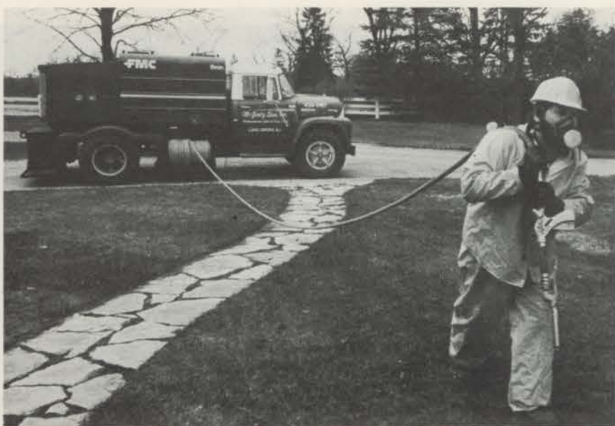
A McGinty worker pulls a spray hose onto a job site.
