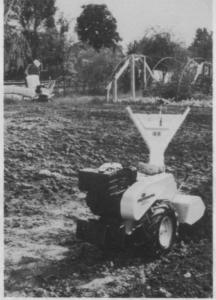
turning. Three-step chain reduction drive uses the Briggs and Stratton industrial engine efficiently: power flows directly from the engine to the chain drive for quick response. The tiller's sixteen self-sharpening, heat-treated tines gives a 26 inch tilling width.
