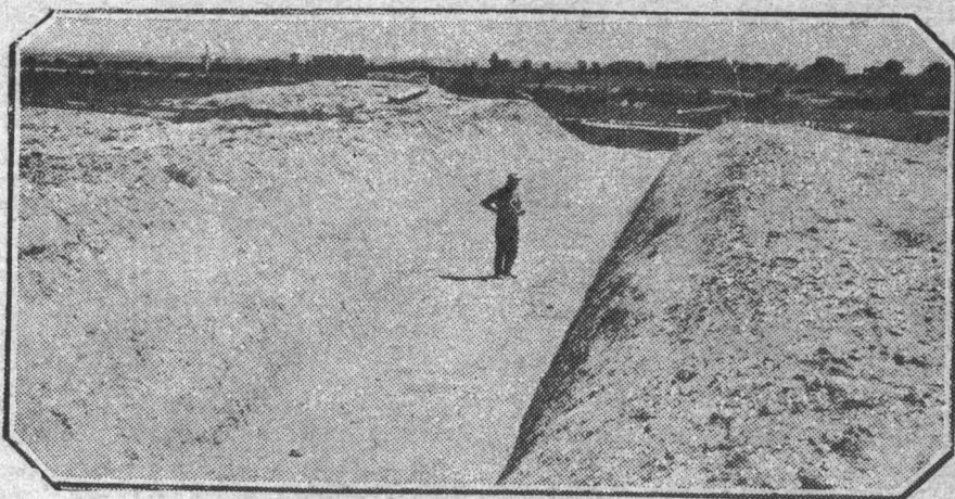
Type of earth silo used in the west. Commercial types of silos are best and do not require so much care in packing, etc.
