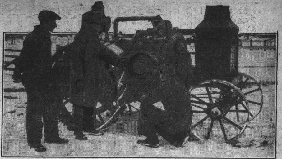
Examining the pulley on an "Oil Pull." The little pulley often gives the farmer his greatest service from the tractor.
