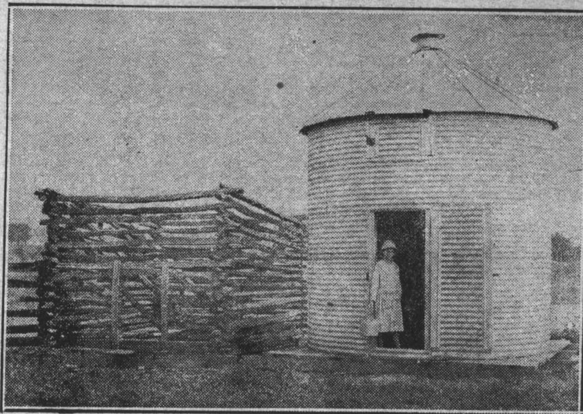
Scene on a corn belt farm showing comparison between the old and new methods of curing corn. The first is exposed to rodents and weather. The second is rat-proof, mould-proof and fire-proof.
