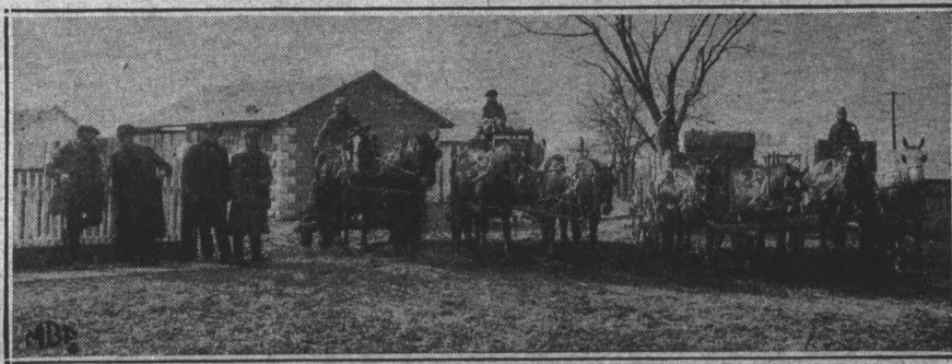
Co-operative scale house and headquarters of one of the local points in Adams County, Illinois.
