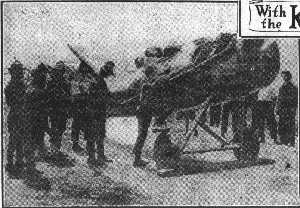
More and more it is being impressed upon the United States Government that airplanes will win the war. Giant factories all over the country are working night and day turning out airplane motors and bodies. The above scene shows mechanics testing out a motor before mounting the wings. There can be chance of a defect in the mechanism. A loose screw, a rusty valve, may mean death to someone.
