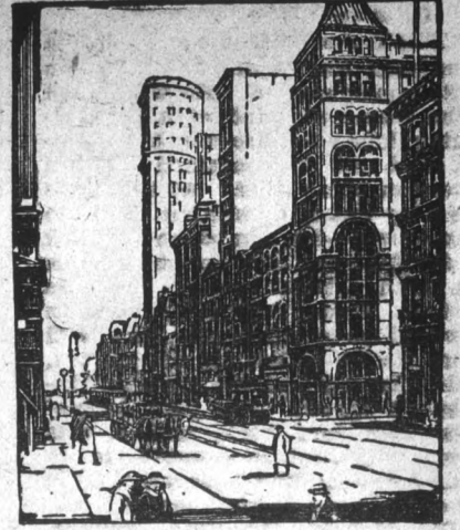
The same scene after the overhead wires were replaced by underground cables.
