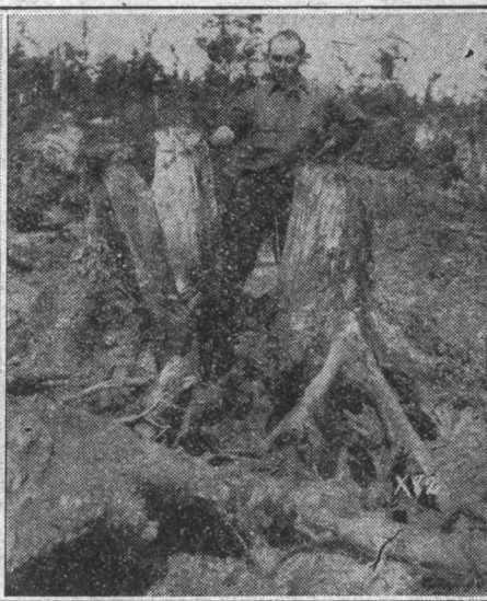
They split 'em like this with dynamite, then yank 'em out with a tractor.
