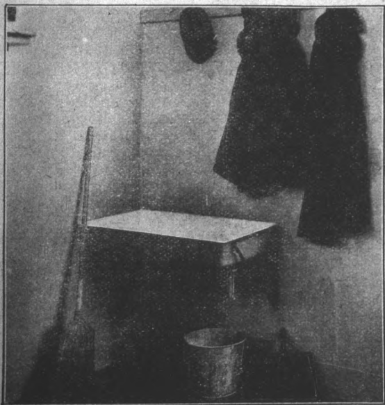
In this case the sink has not been properly installed. In the first place it is placed back in a corner where the light is very poor. No woman would care for a sink located like this one. It should be near a window. Also this sink has an inadequate method of sewage disposal. When the pail is full it is necessary to carry it outdoors making many steps that are not necessary.
